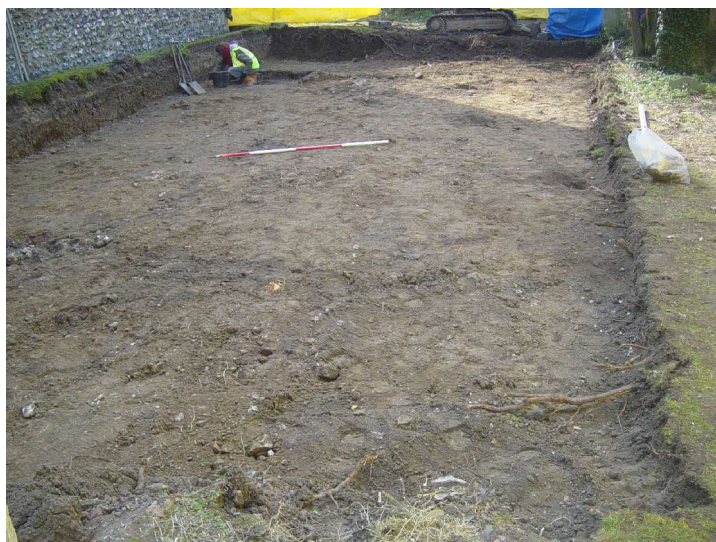
Fig 15 View of the initial stages of the site reduction and hand clearance Phase 1 works, looking west from the corner of the bell tower. The long shadow cast over the site by the nave is evident in this photograph, but even in the best light and after careful hand cleaning, no clear grave cuts were discernable in the homogenous upper layer denoted [103].
