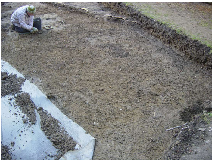
Fig 19 A member of ODAS assisting with the hand clearance in the north east corner of the site. It was in this area that the remains of a font were discovered, the design on the greensand accords with published records of the old church font and the font was lifted by ODAS and will be displayed in the churchyard.
