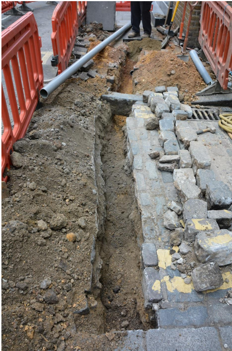
Figure 7: Section of trenching crossing Spital Yard. Facing E. No scale.
