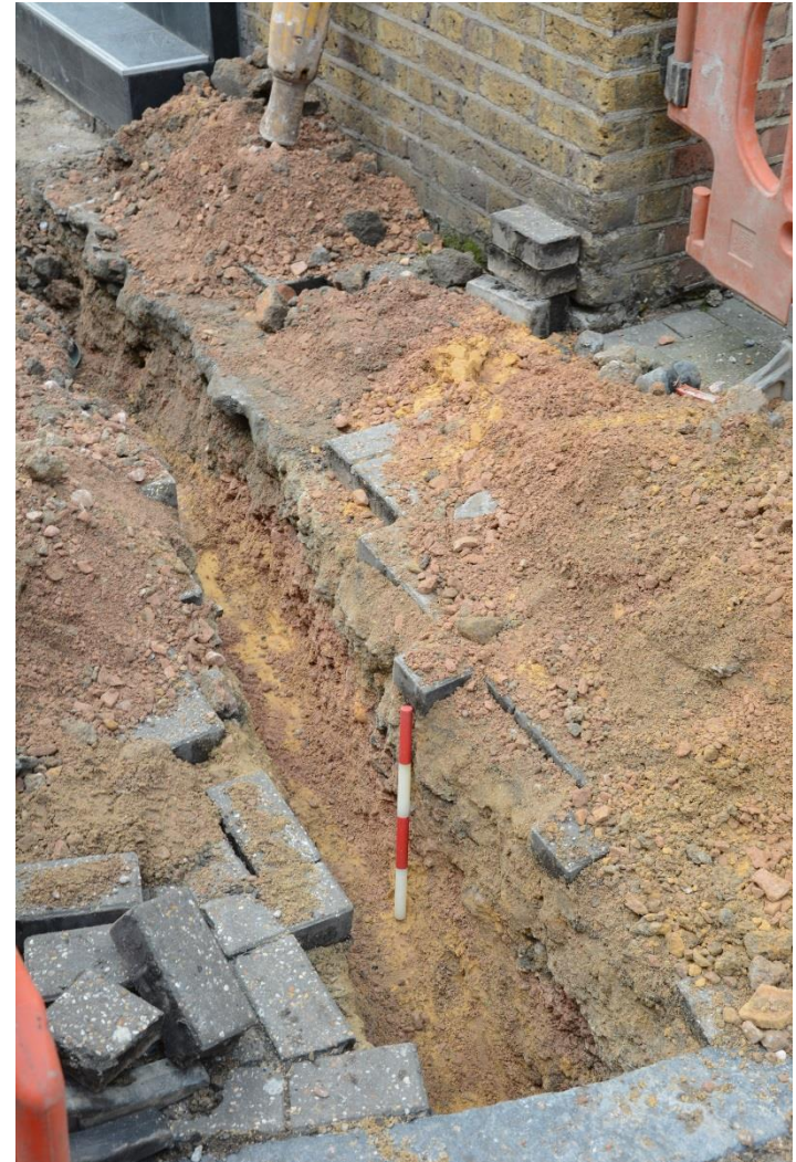
Figure 4: Detail of north facing section. Facing SE. Scale 0.4m.
