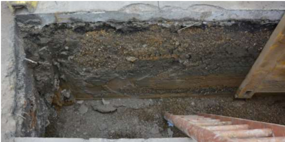
Fig.4: South-facing section through west end of trench, 17.02.16. Facing N
