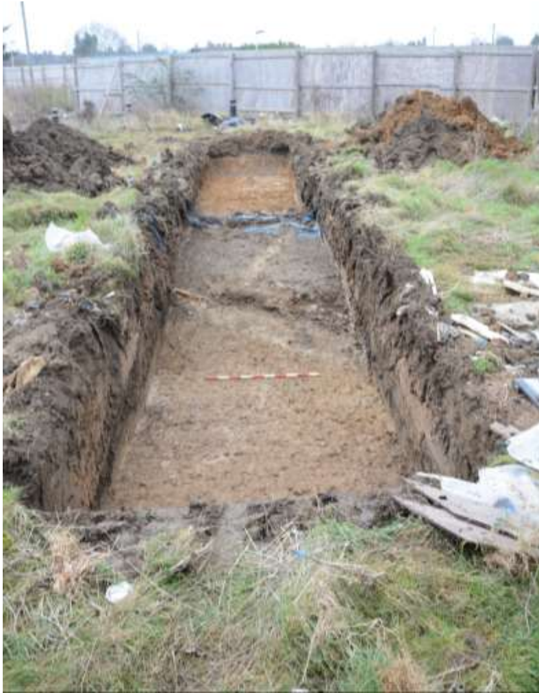
Fig. 20: Overview of Trench 4, showing existing services and natural gravels at the southern end. Facing SSE. Scale 1m.
