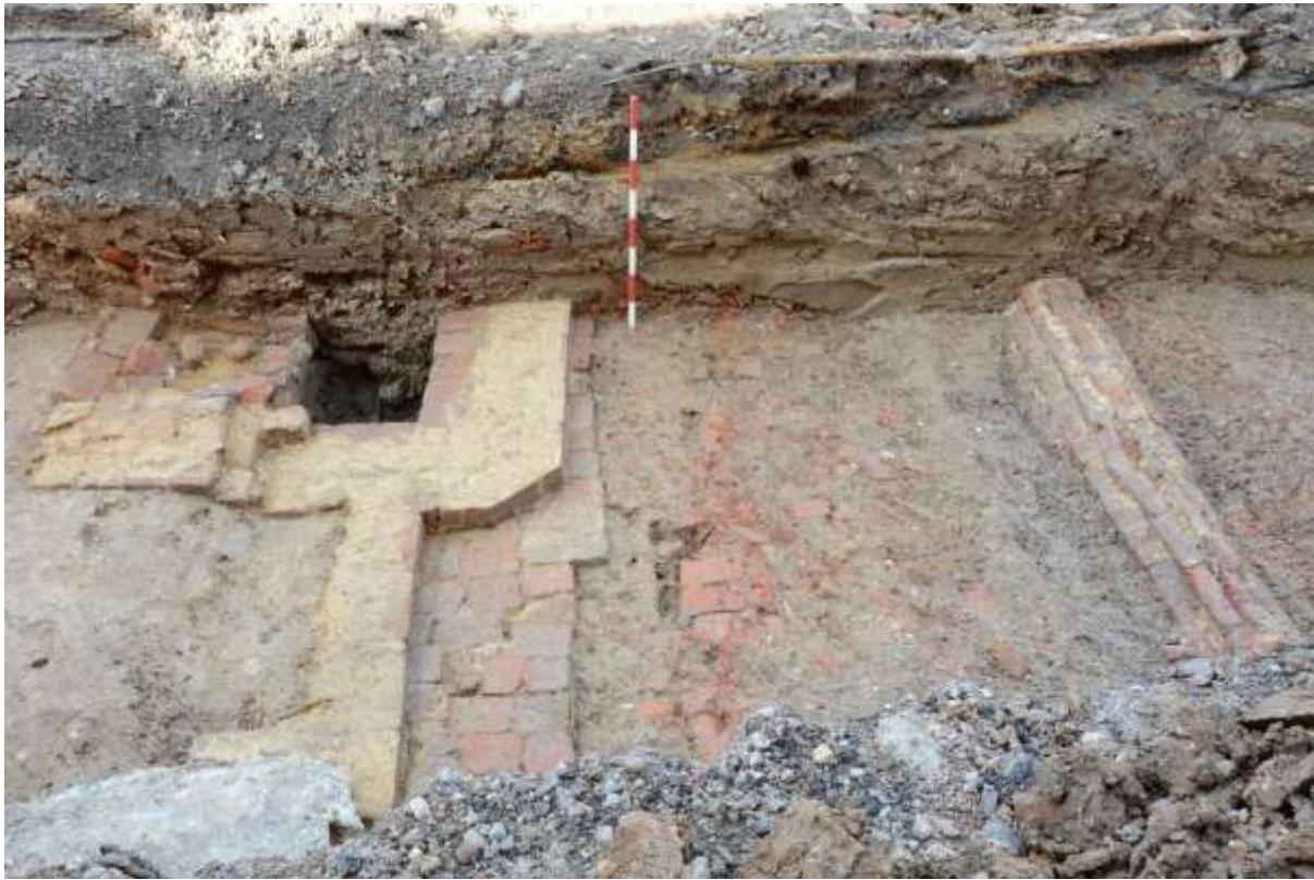
Fig.20: SW section of Trench 2 showing the main masonry features, facing SW (0.8m scale)
