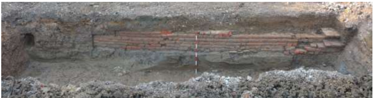
Fig.17: View of southern section with brick wall [8], facing SE (1m scale)
