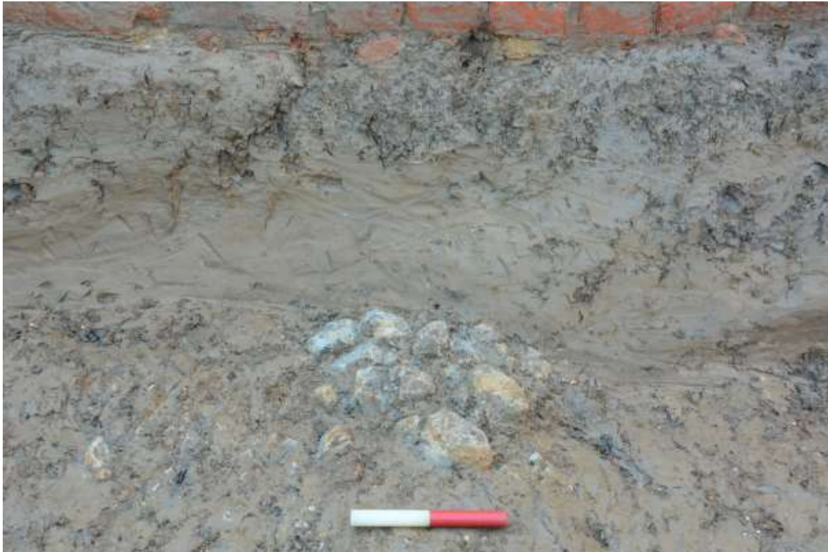
Fig.18: Detail of one of four possible stone building pads [10], facing SW (0.2m scale)
