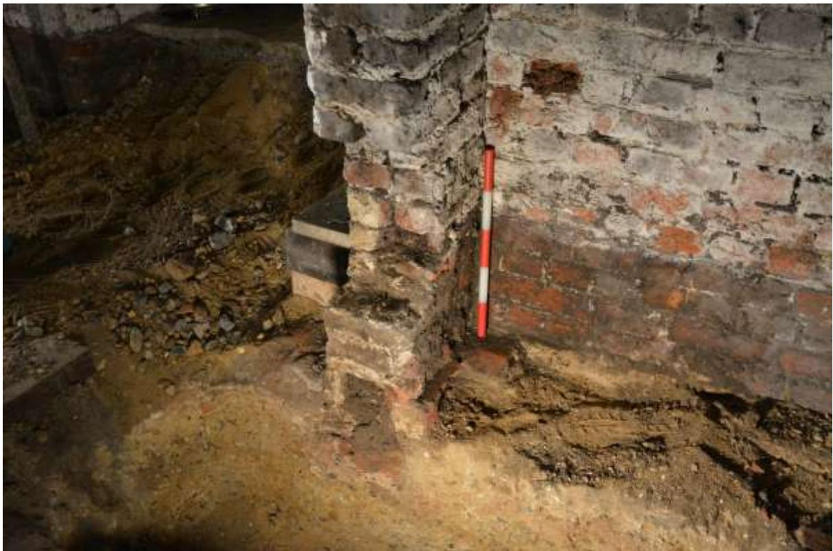
Fig.9: Main cellar dividing wall and later addition projecting and overlying / truncating cellar floor, facing E, 0.50m scale
