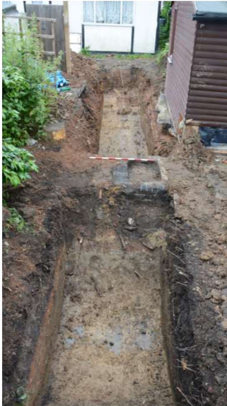
Fig. 14: View of full length of trench 2, facing SW, 1m scale
