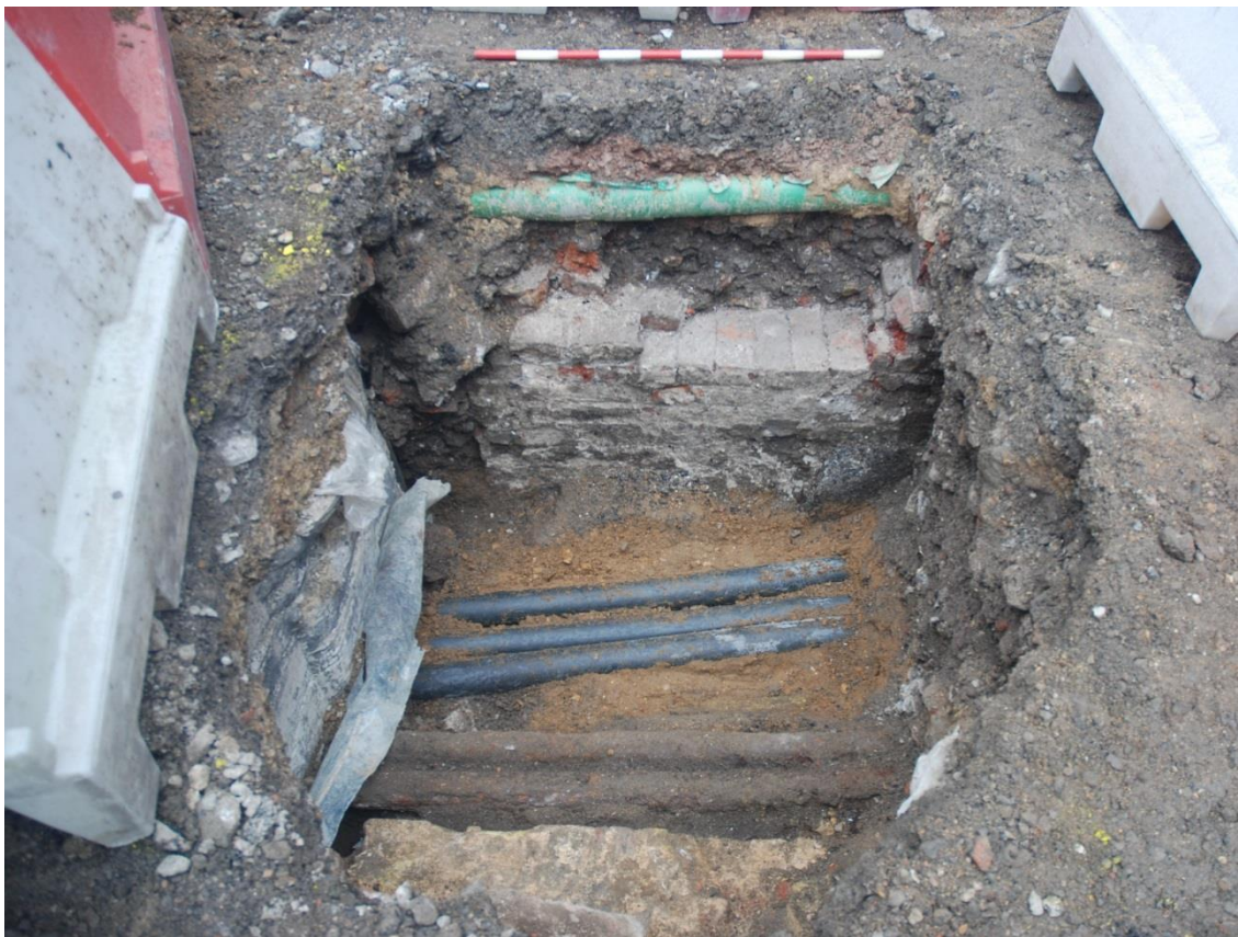
Figure 13: Overview of Trench 3. Facing W. Scale 1m.
