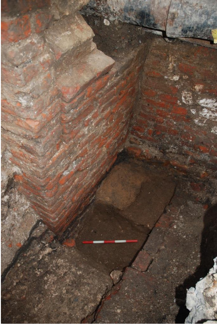
Figure 5: Brick structure exposed by Compass in 2014, facing SW, post removal of brick floor. The 50cm scale rests within the robber / construction cut for structure [6]. The remnants of the City wall, [15], are visible as a block of mortared masonry in the bottom left of frame. The scale rests on top of, and adjacent to Roman deposit (16), towards the corner of the later structure.
