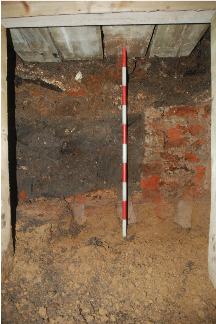
Figure 9: Wall [16] see in the north facing section of the N-S spur, to the right of a possible pit feature (18). Facing S. Scale 1m.
