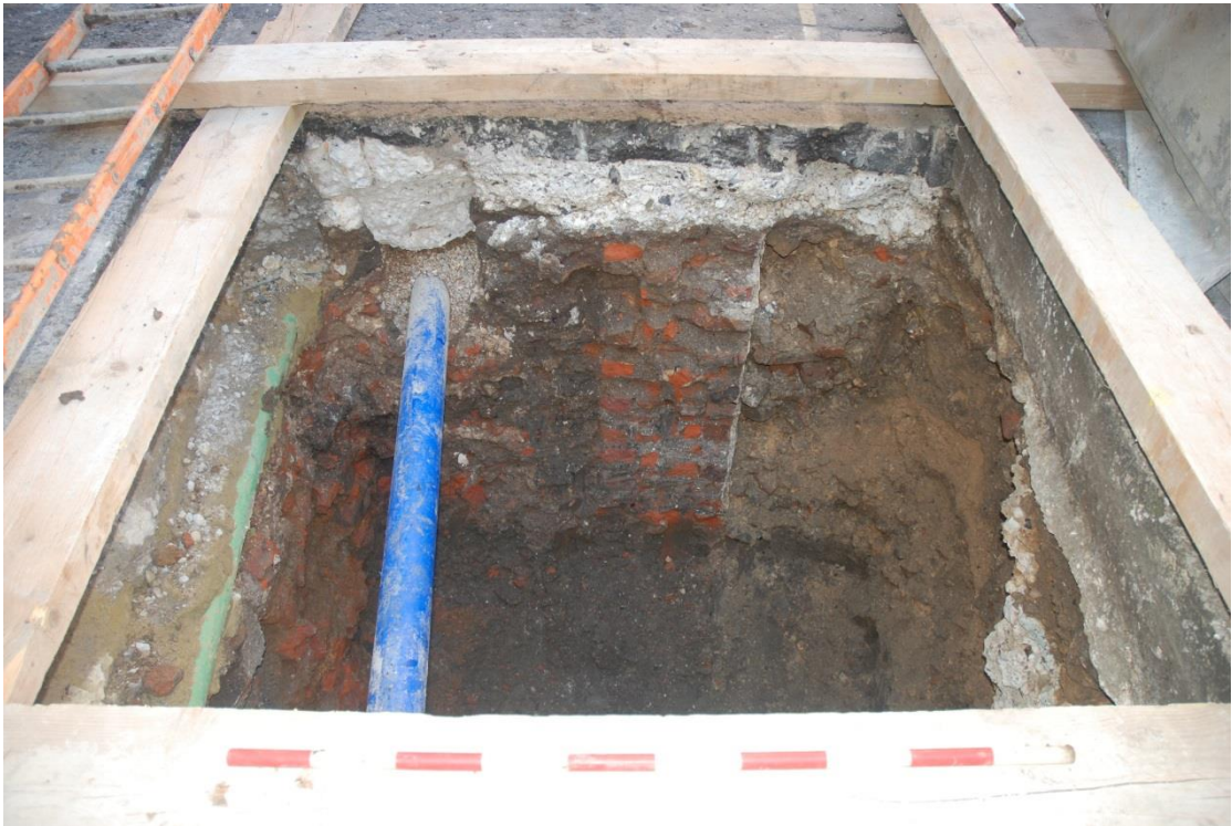
Figure 6: Upper 2m of Post-medieval stratigraphy, including wall [4], backfill to north (9) and fill (5) to south. Facing W. Scale 1m.
