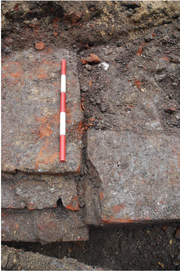
Figure 14: Detail of the relationship between [26] (left) and [28]. Scale 0.5m.
