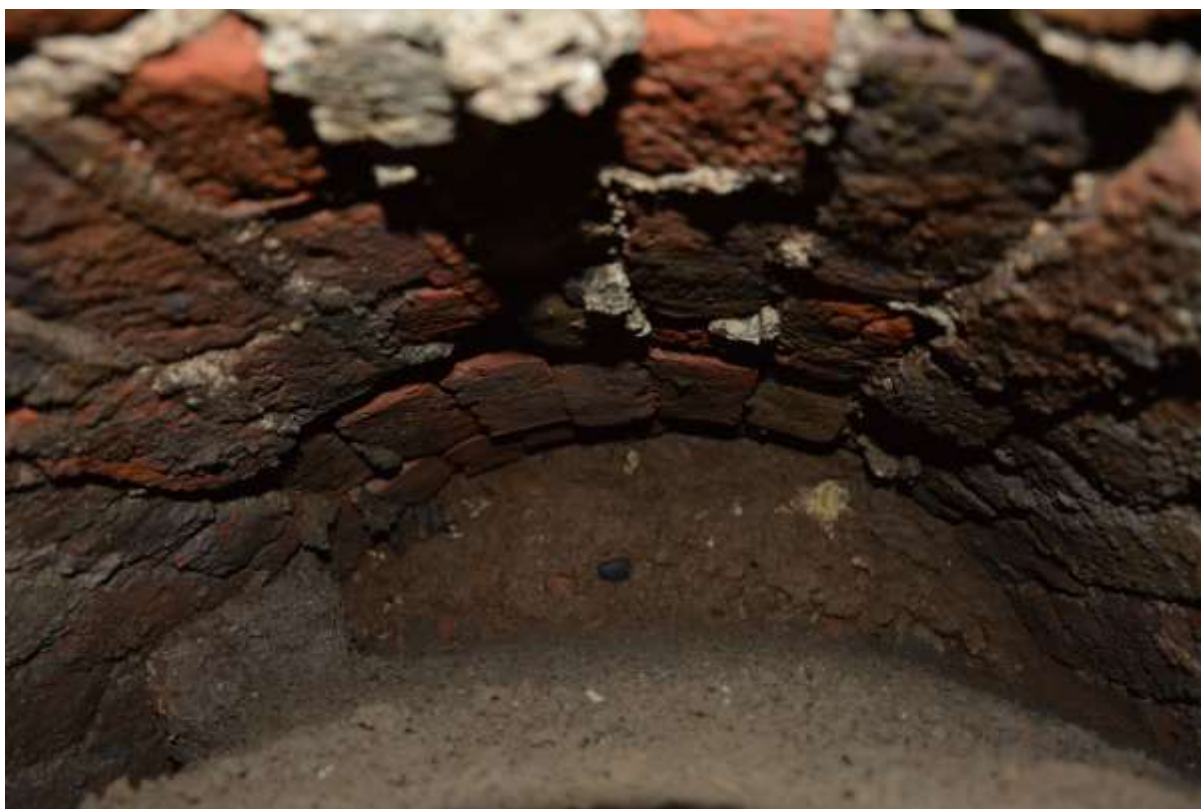
Fig.20: Internal shot of drain [1106] facing east, showing silting (1105)
