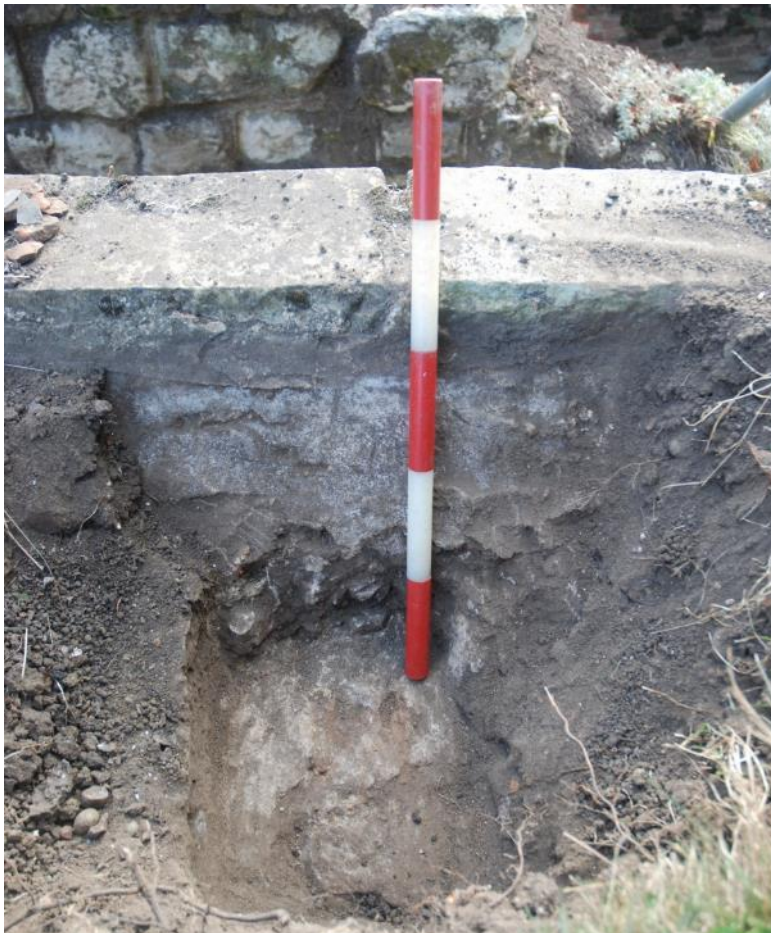
Figure 13: Pit 12, east end of balustrade. North facing section, showing the sloping rear-side of the wall, coming down on to a wider concrete footing. Facing S. Scale 0.5m.
