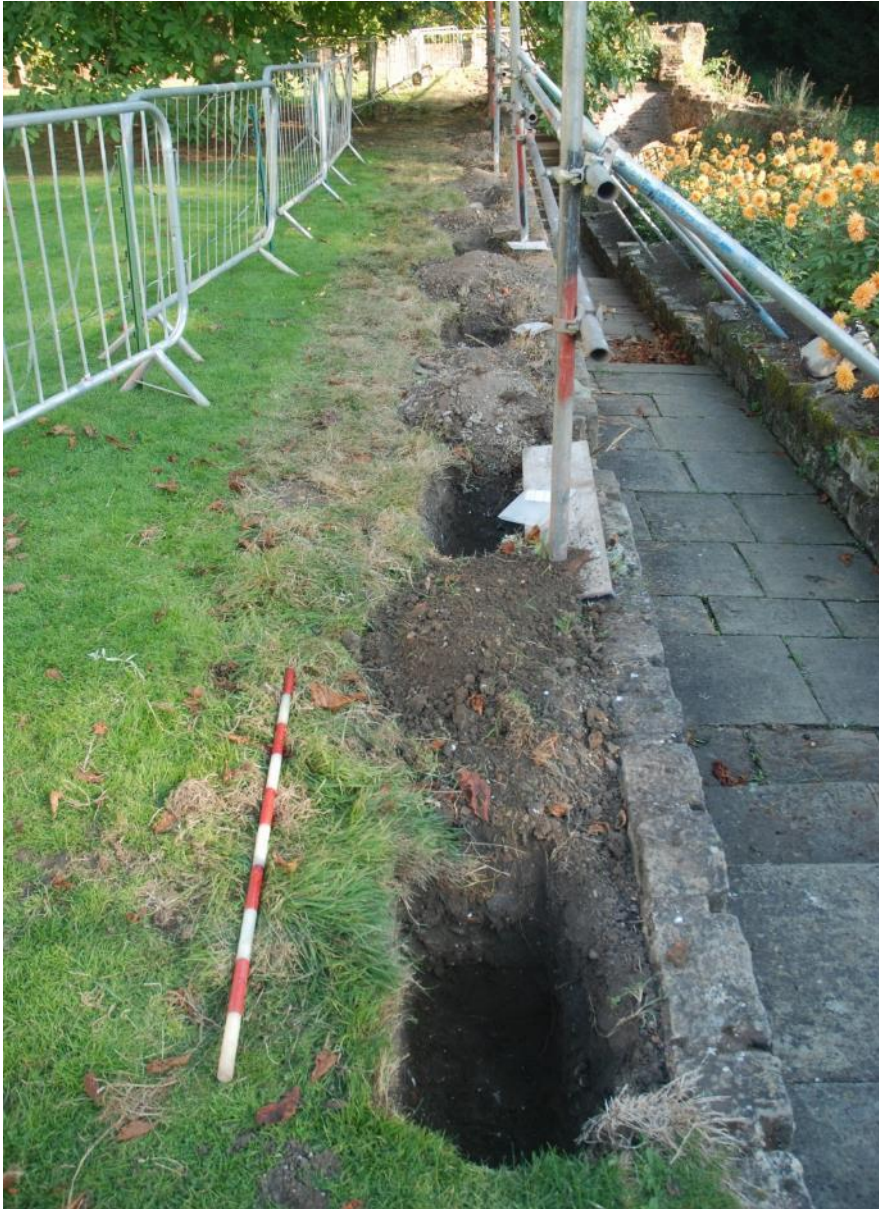
Figure 9: Completed trenches following the removal of the balustrade. Photograph taken from the west end, facing E. Scale 1m.
