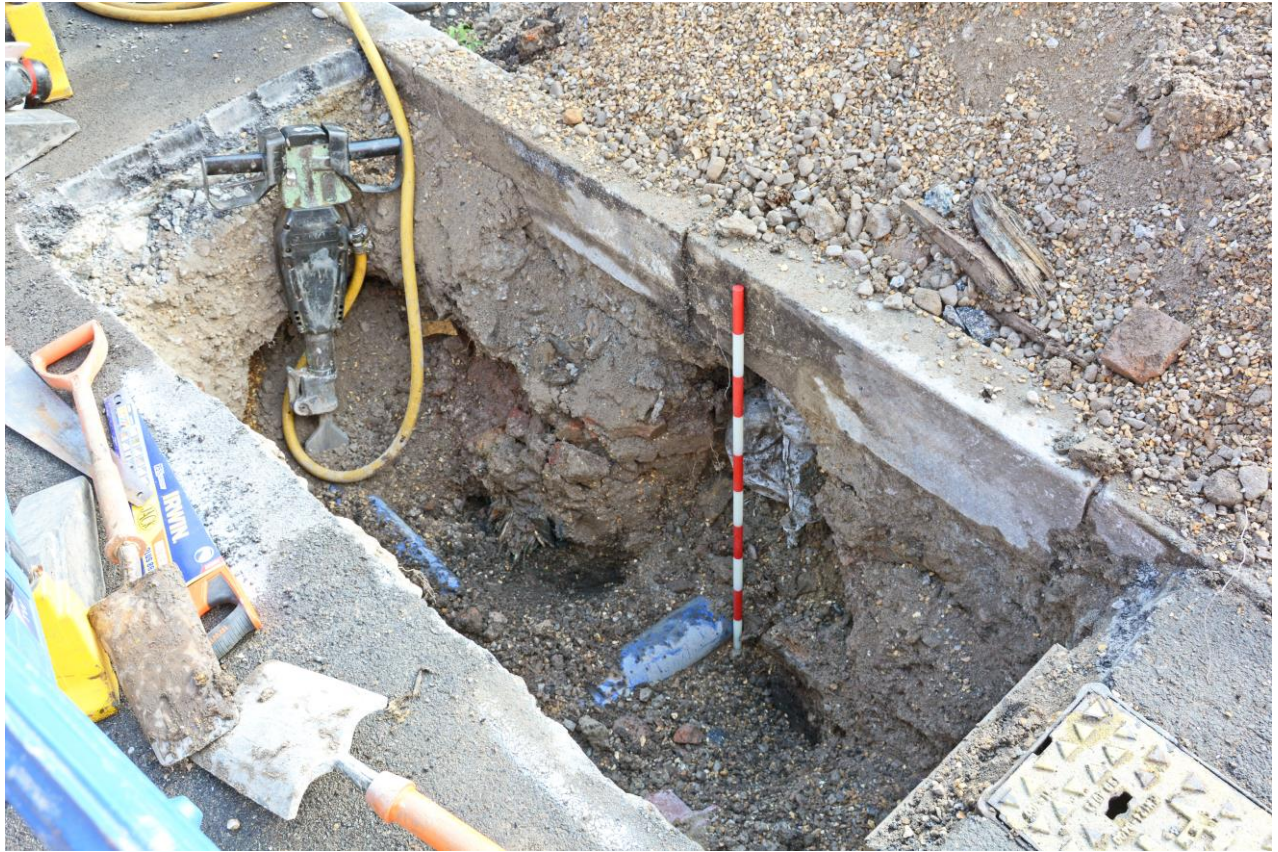
Fig.2: View after excavation of the trench looking east (1m scale)
