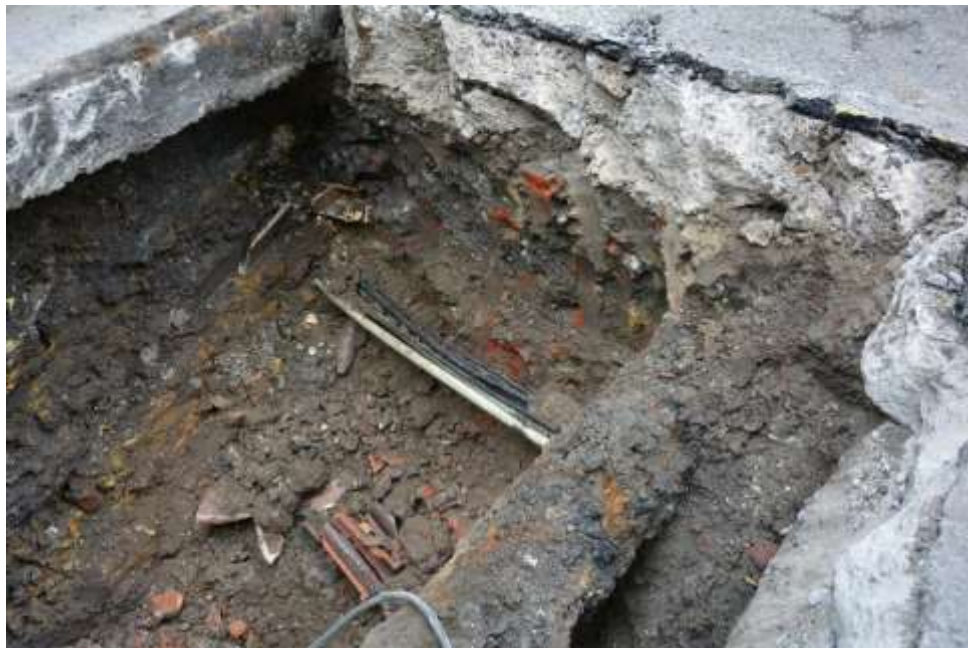
Figure 10: View of services cut into (6), facing SW
