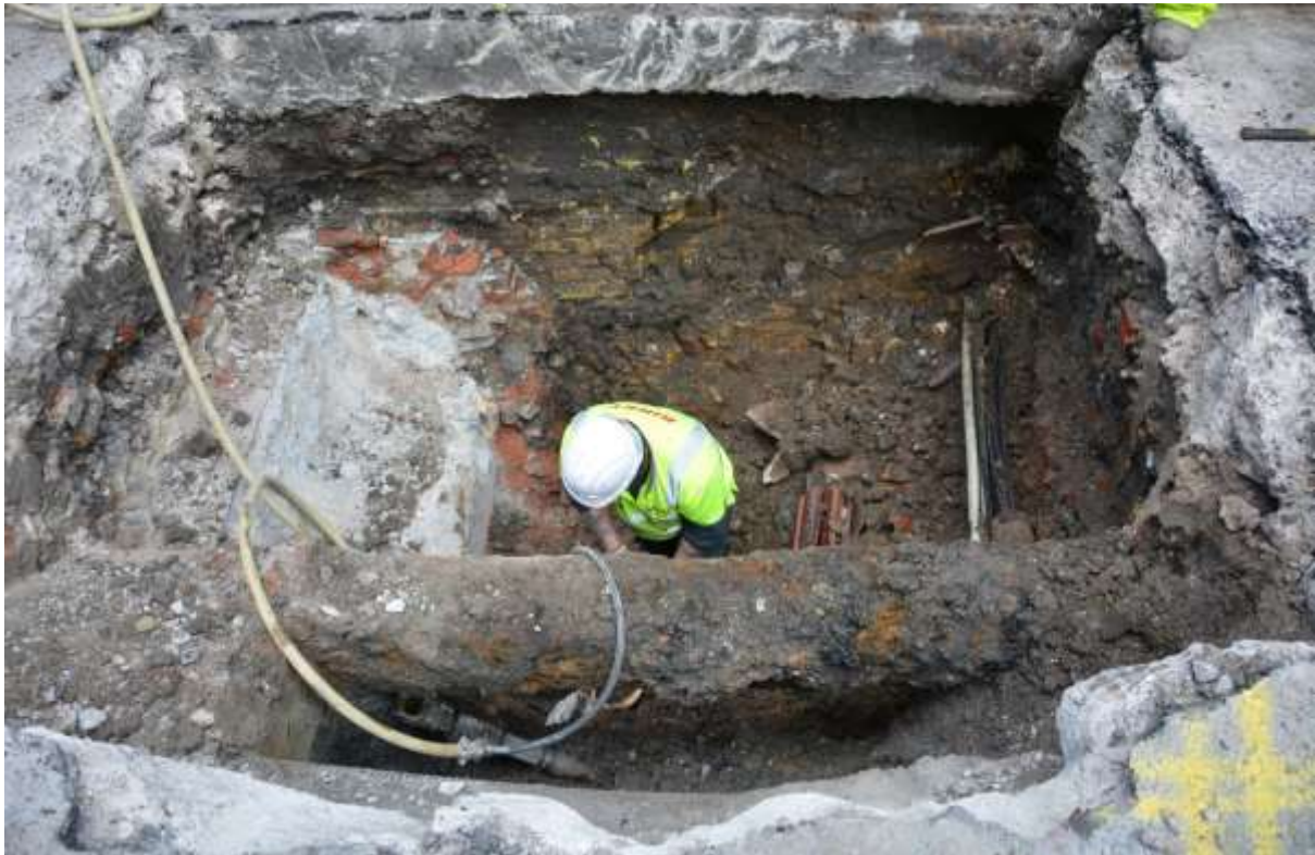
Figure 9: View of yellow stock brick wall, facing SW. Unfortunately no direct access to the drop shaft was attainable at this time due to safety concerns
