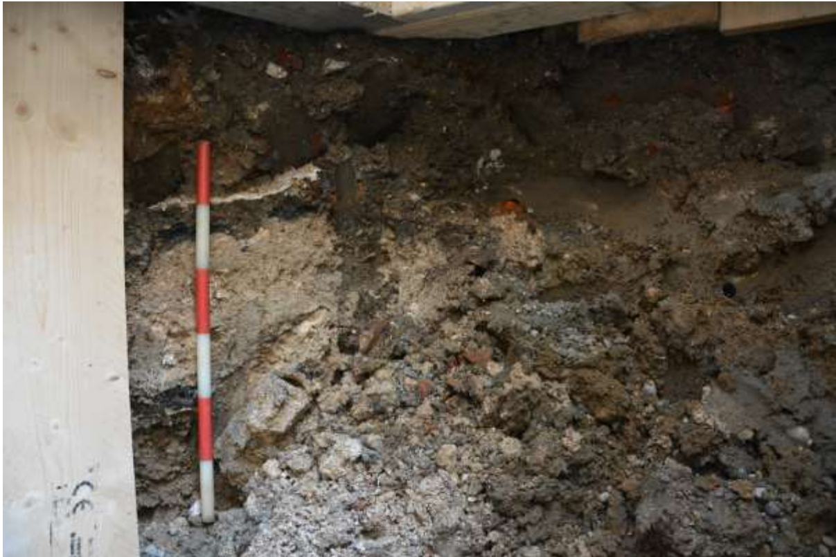
Figure 15: View of NE corner of NW section showing isolated mortar deposit, facing NNW, 0.6m scale
