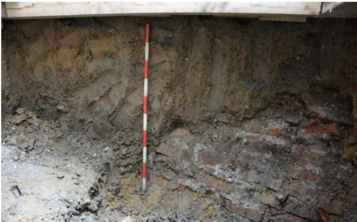
Figure 17: Wider view of disused red stock brick sewer/culvert [9] in NE section, facing NE, 1m scale
