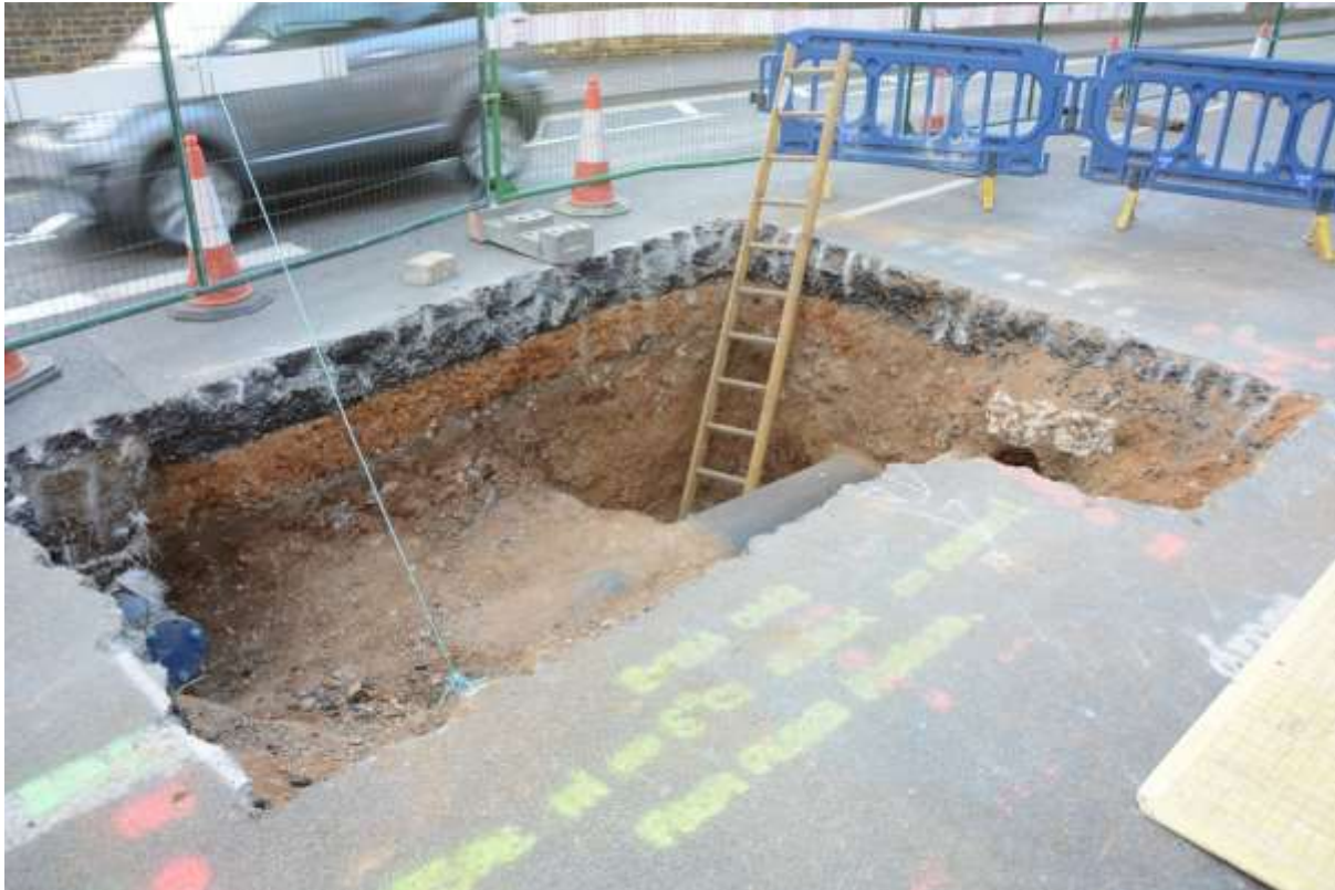
Fig.8: Trench facing southeast
