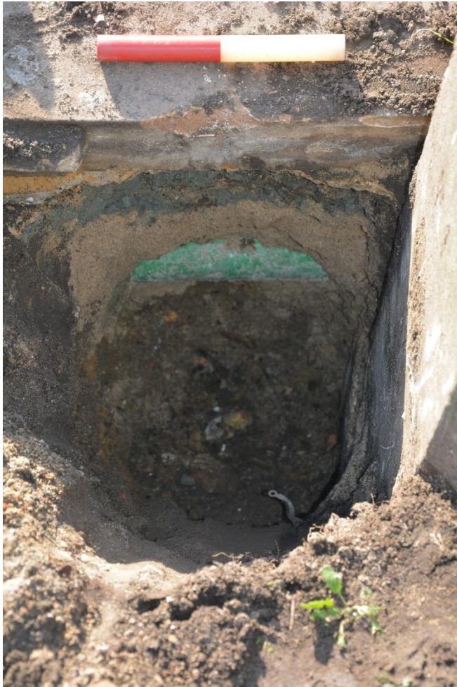
Figure 11: E: Stratigraphy in the westernmost pit: Paving slabs (8) above concrete bedding layer (9), sealing a service cut [6] / (7) and backfill (2). Facing S. Scale 0.2m.
