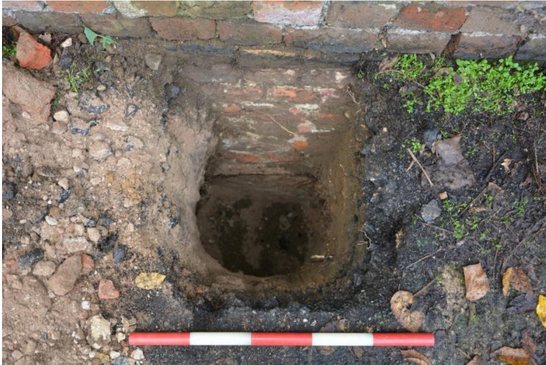
Figure 14: TP3 - exposed footings, significantly deeper than those exposed in TP1. Facing W. Scale 0.5m.
