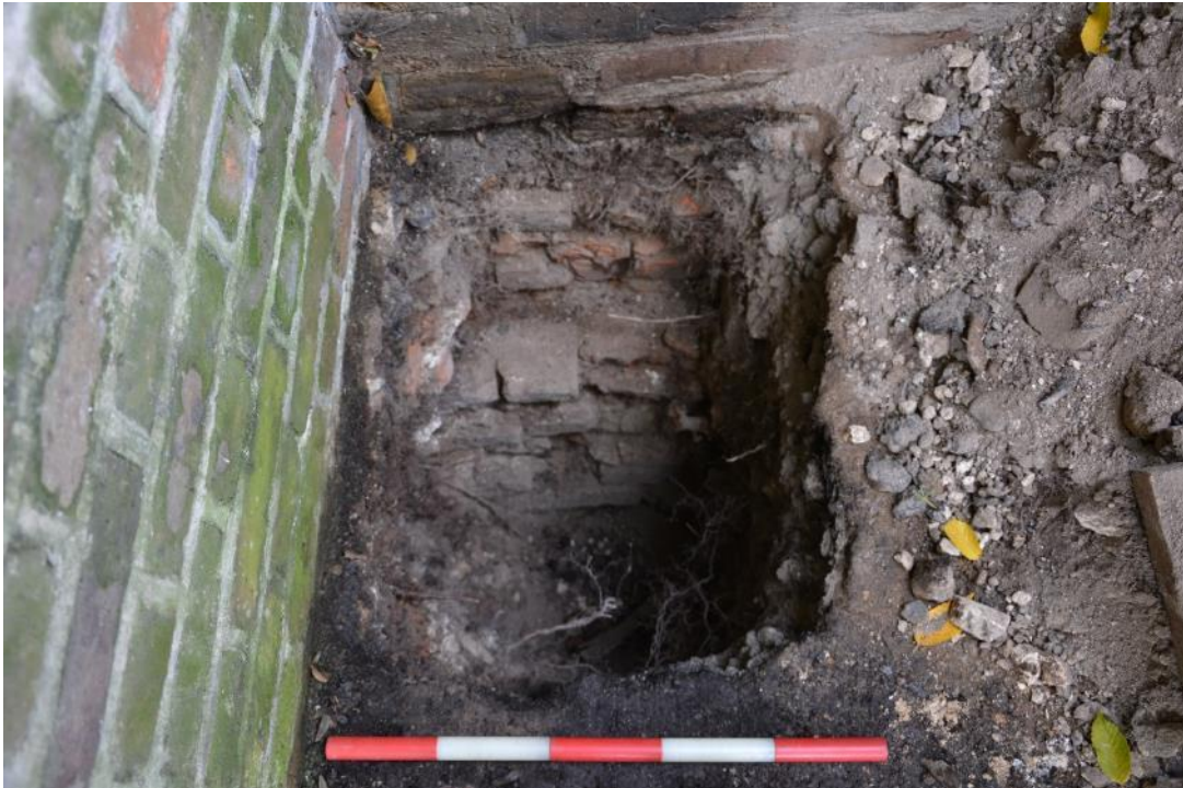
Figure 18: TP5 - extremely loose and fragmented foundations of the party wall. Facing W. Scale 0.5m.
