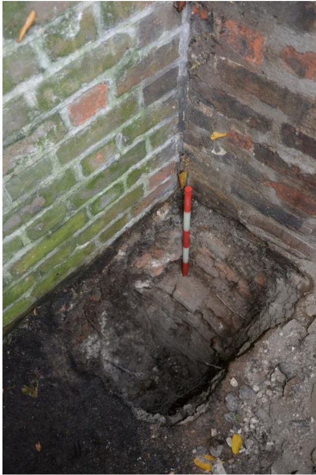
Figure 19: TP5 - crumbling foundations and rubble abundant backfill below macadam surface. Facing SSW. Scale 0.5m.
