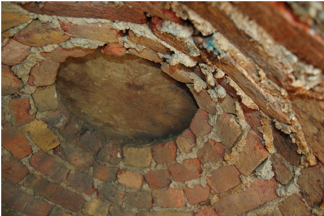
Fig 6 Photograph of the inside of the domed roof and slab capping of the well in Trench 1
