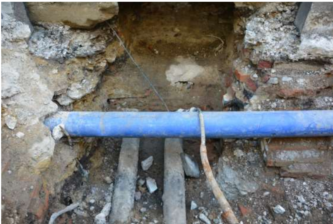
Figure 28: View of north eastern side of [203] and services, facing NE
