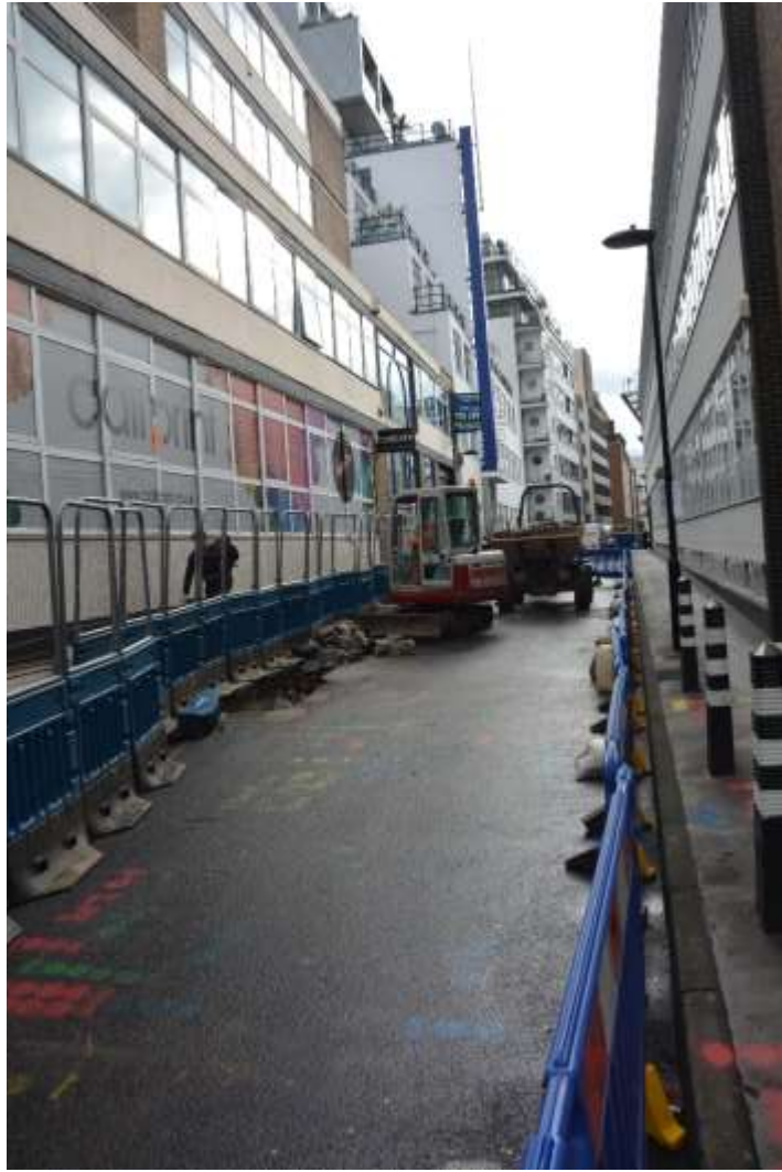
Figure 14: View of trench on Saffron Hill, facing SW
