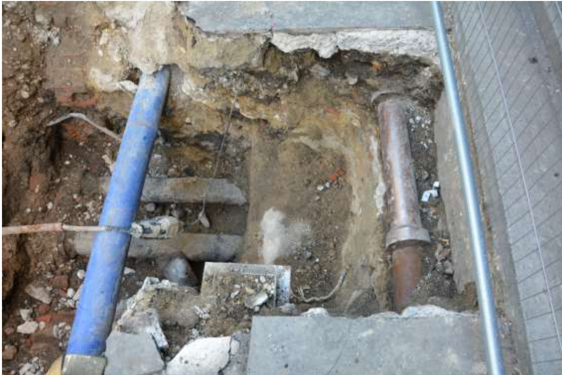
Figure 26: View of the ceramic pipe in trench 2, facing NW
