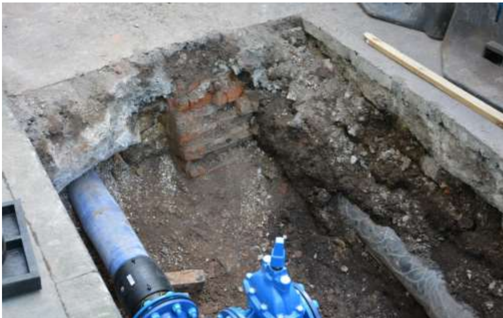
Figure 25: Oblique view of the NW section of the trench, facing N
