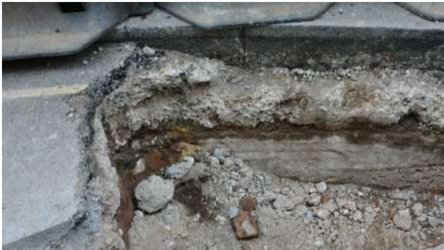
Figure 23: View of the end of the final bay of [104], facing NE
