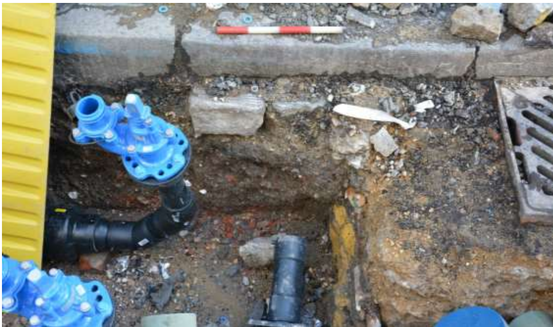
Figure 30: Section of trench 3, facing NE, 0.4m scale
