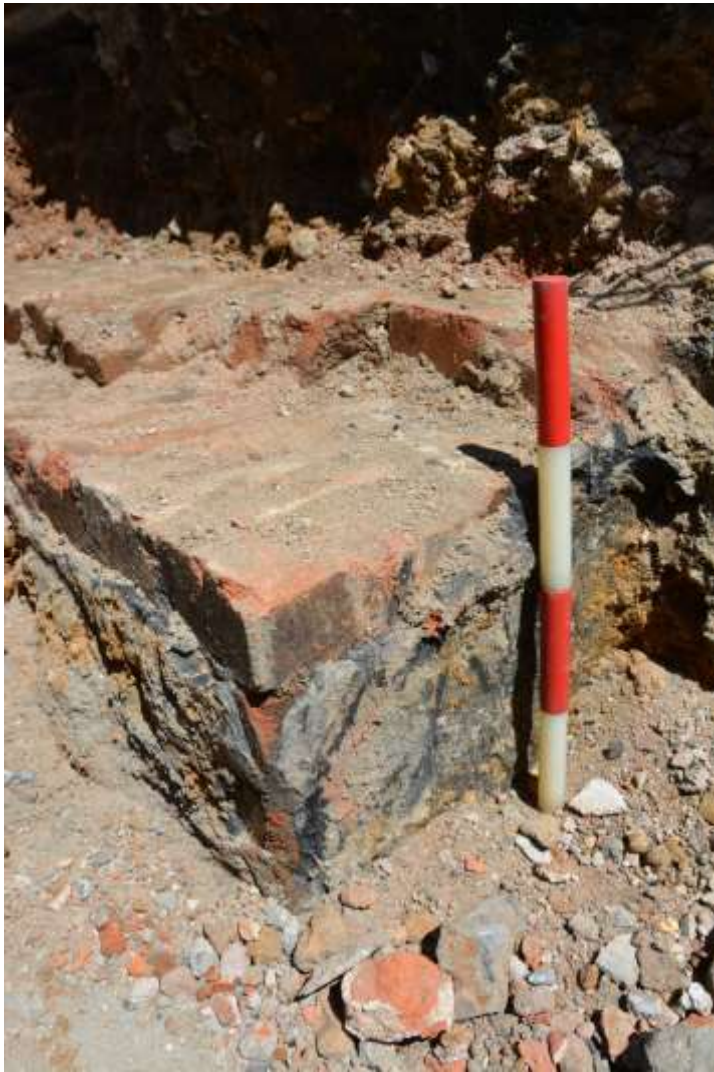
Figure 47: Detail of the rendered side of [905], facing NE, 0.4m scale
