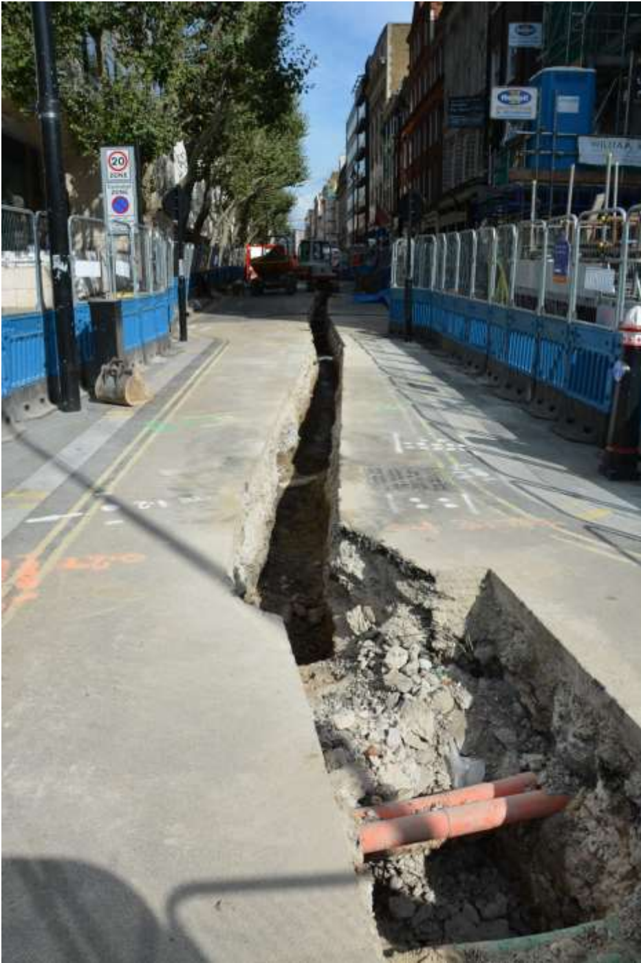
Figure 51: View of trench 10 from Holborn Circus, facing NW
