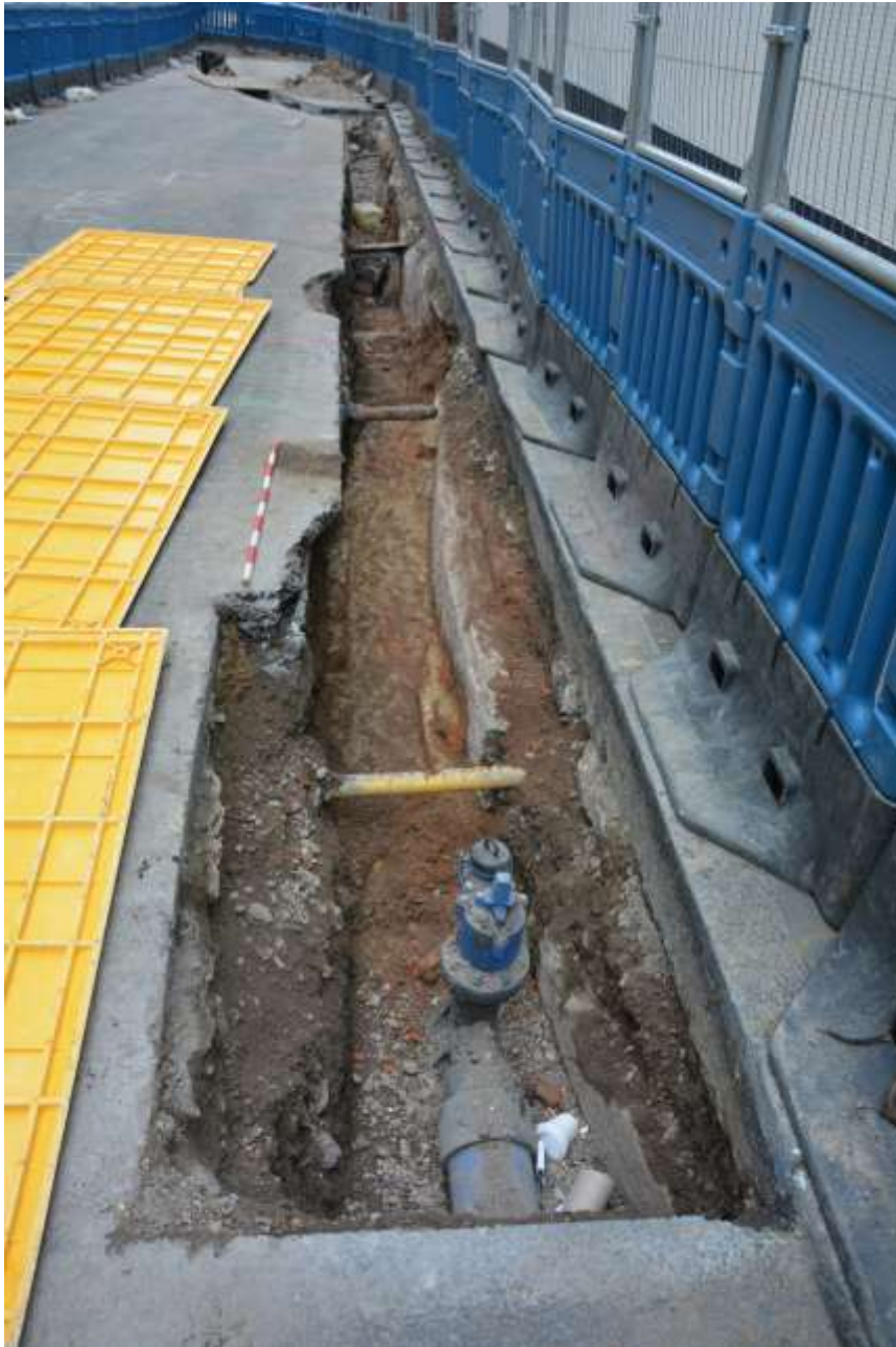
Figure 17: View of the extent of trench 1, facing NW, 1m scale
