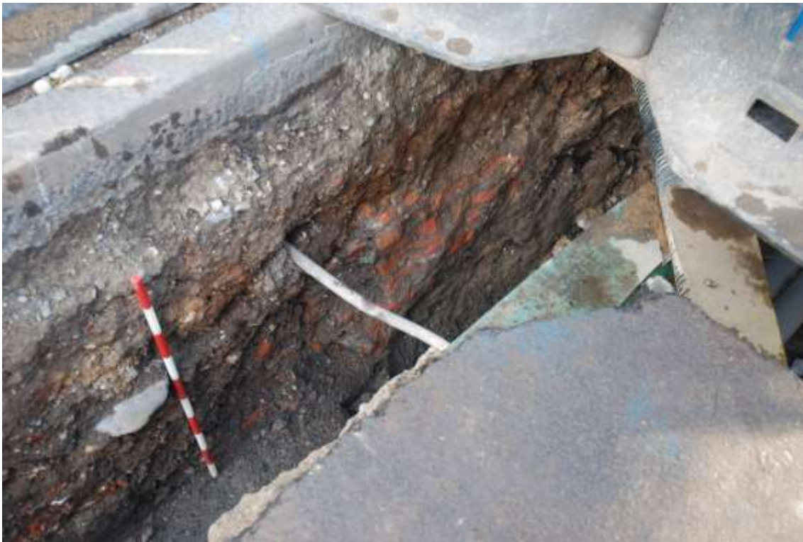
Figure 34: Oblique view of wall [504], facing NE, 1m scale
