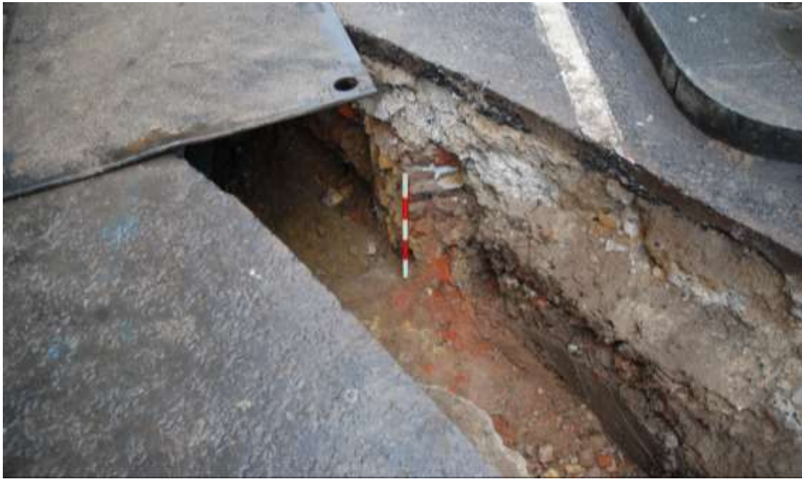
Figure 62: Part of yellow and red stock brickwork [1403], facing SW, 0.5m scale
