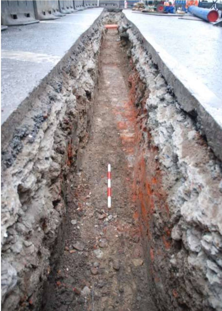
Figure 61: View of [1402], facing N, 0.5m scale
