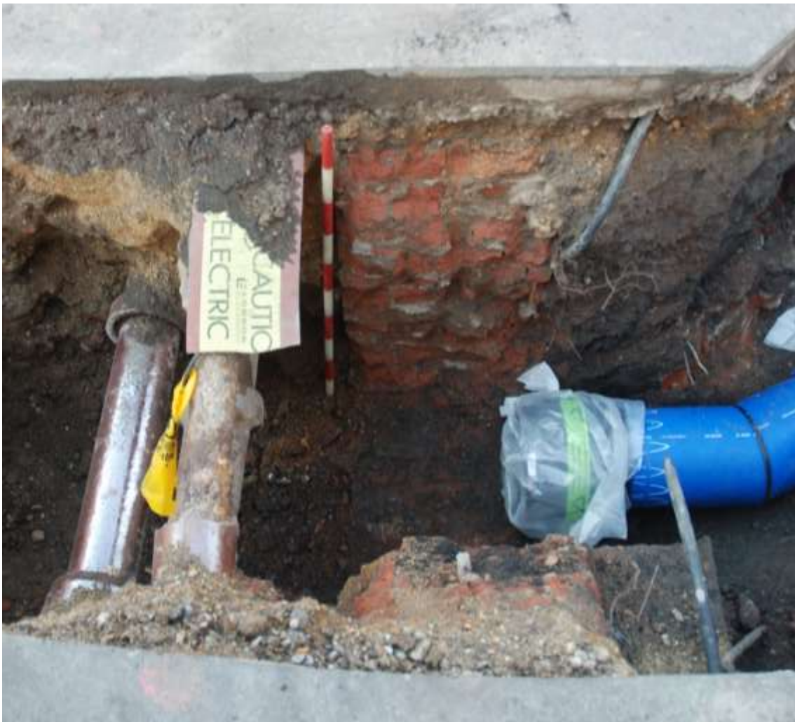
Figure 58: View of post-medieval brick wall [1304], facing W, 1m scale
