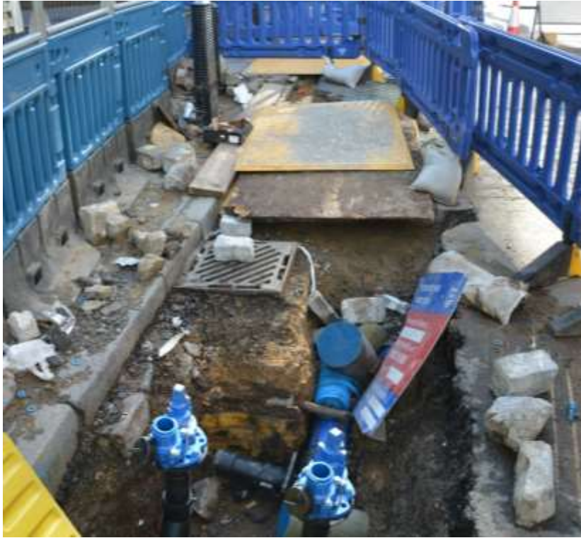
Figure 29: General view of trench 3, facing SE
