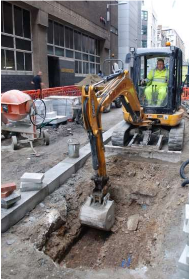
Figure 9: Machine excavating pit three. Facing NW. No scale.
