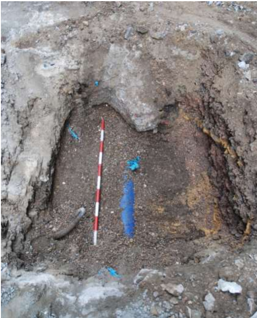
Figure 7: Tree pit two showing water main [5]/(6). Facing NE. Scale 1.0m
