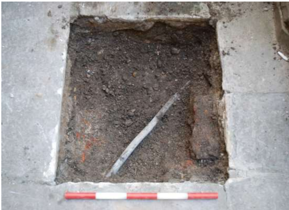
Figure 5: Pit 5, showing post-medieval backfill below the existing paved surface and water pipe. Facing N, scale 0.5m.
