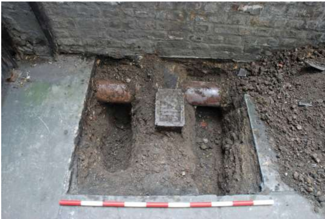
Figure 7: Pit 8, showing backfill surrounding ceramic pipe and associated metal drain. Facing S, scale 1m.
