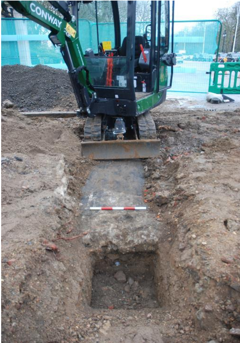
Figure 9: Slab beneath walkway on southern side of The Mall. Taken to be a previous road surface or similar. Facing SW, scale 0.5m.
