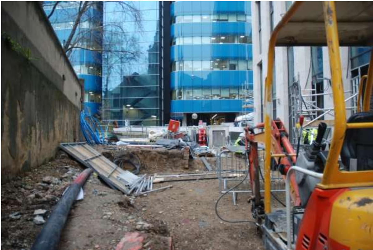
Figure 22: View of St Botolph Row during general ground reduction, facing NE
