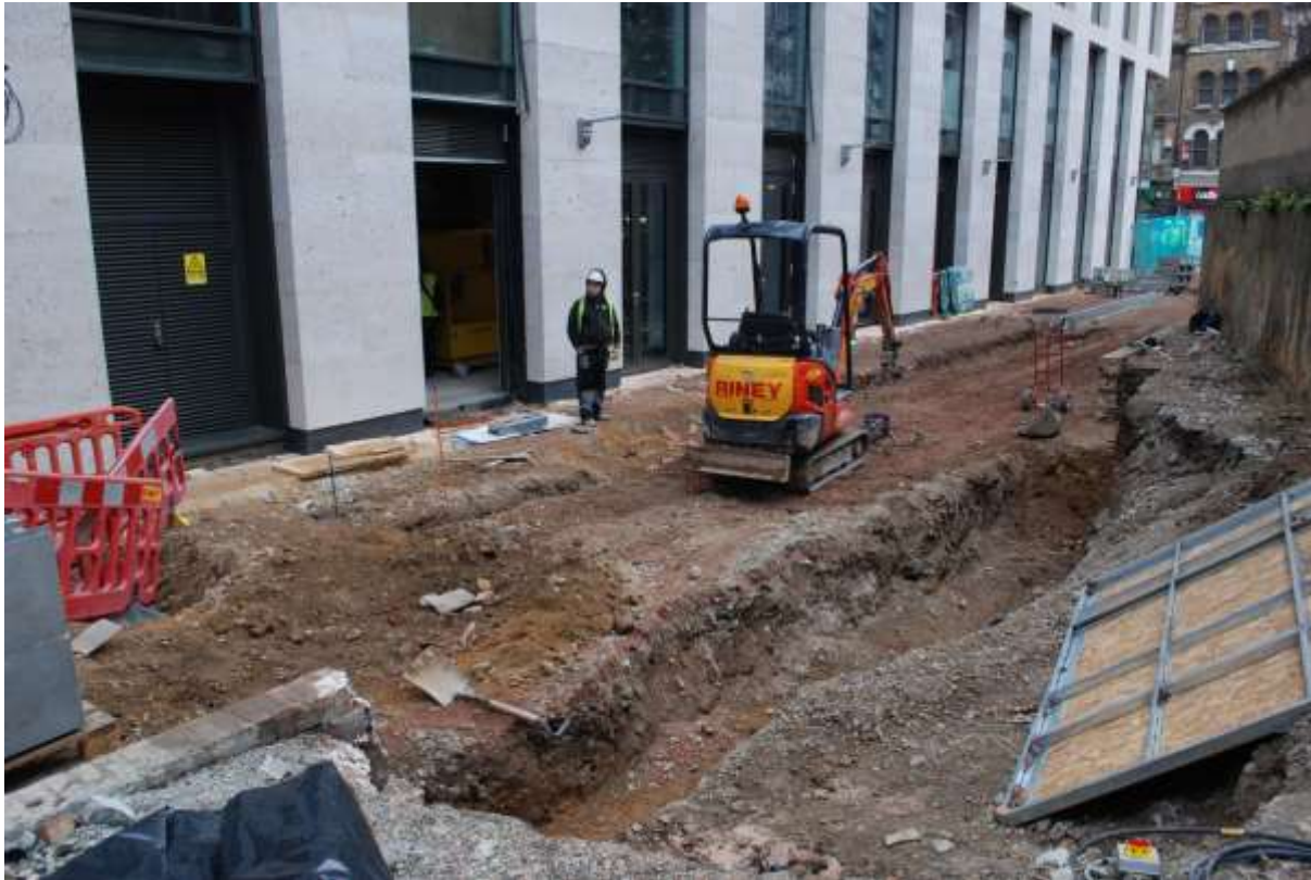
Figure 35: Oblique view of trench 2, facing SE
