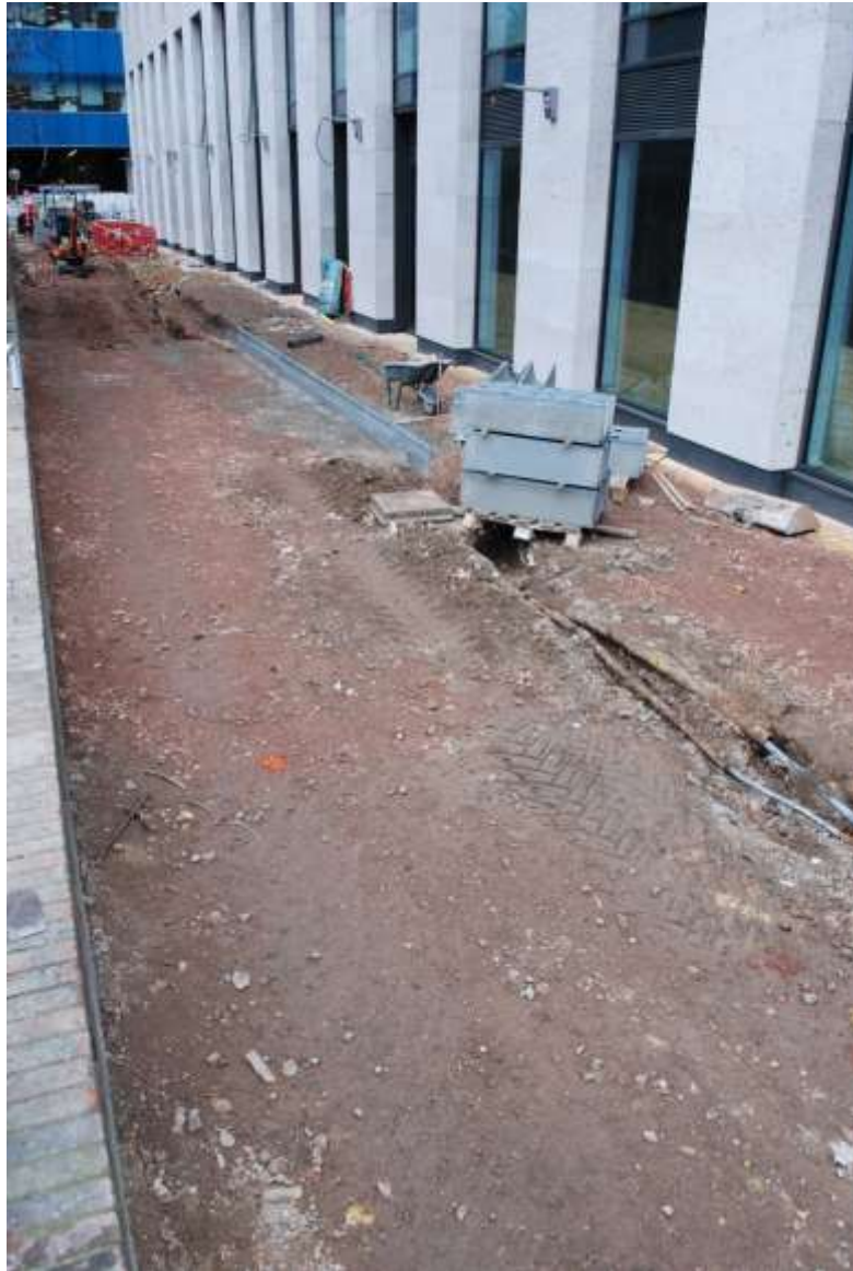
Figure 34: View of the extent of trench 1, facing N
