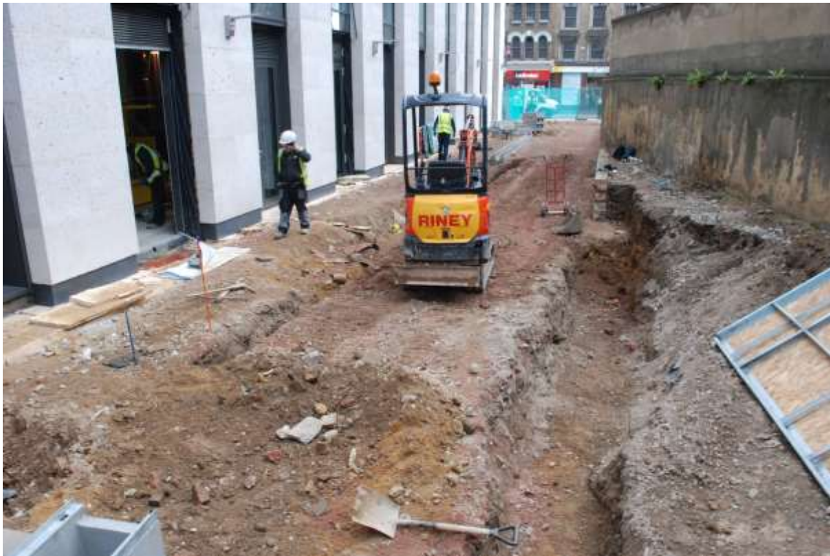
Figure 27: View of trench 1, facing E
