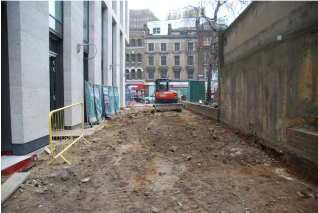
Figure 21: View of St Botolph row during general ground reduction, facing SE
