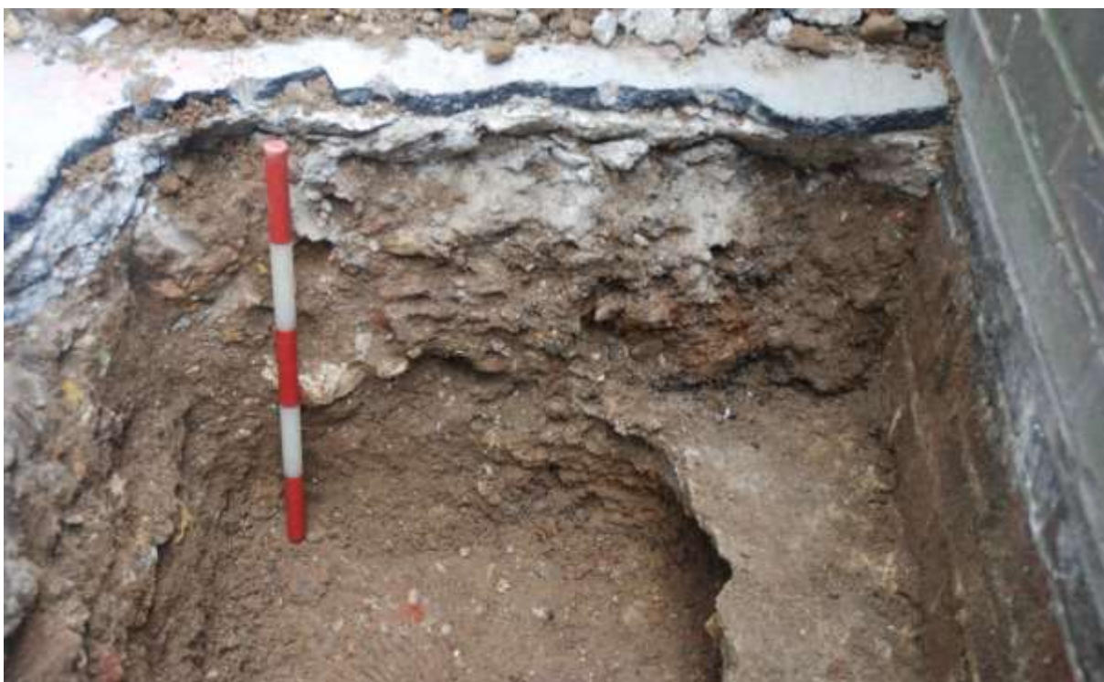
Figure 19: Trial hole 2 SE section facing SE, 0.5m scale
