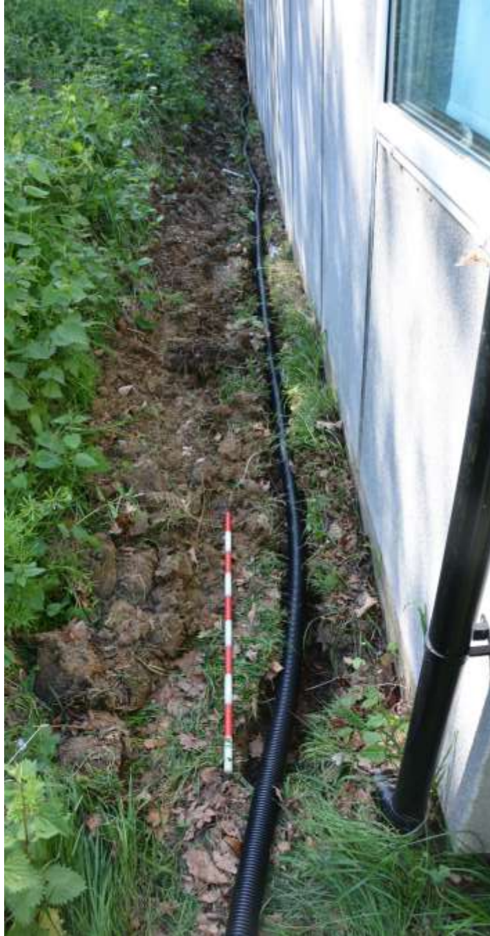
Figure 17: Portion of cable trench behind hutted classroom facing SE, 1m scale
