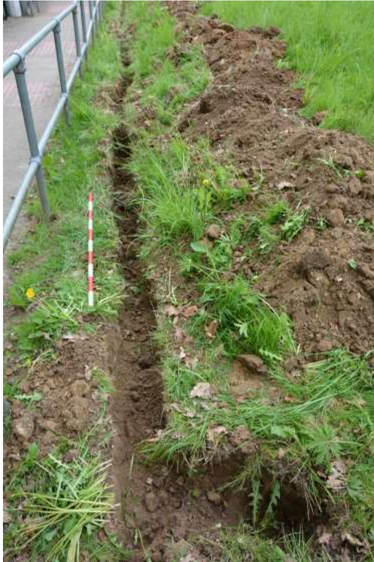
Figure 12: View of cable trench facing SW, 1m scale
