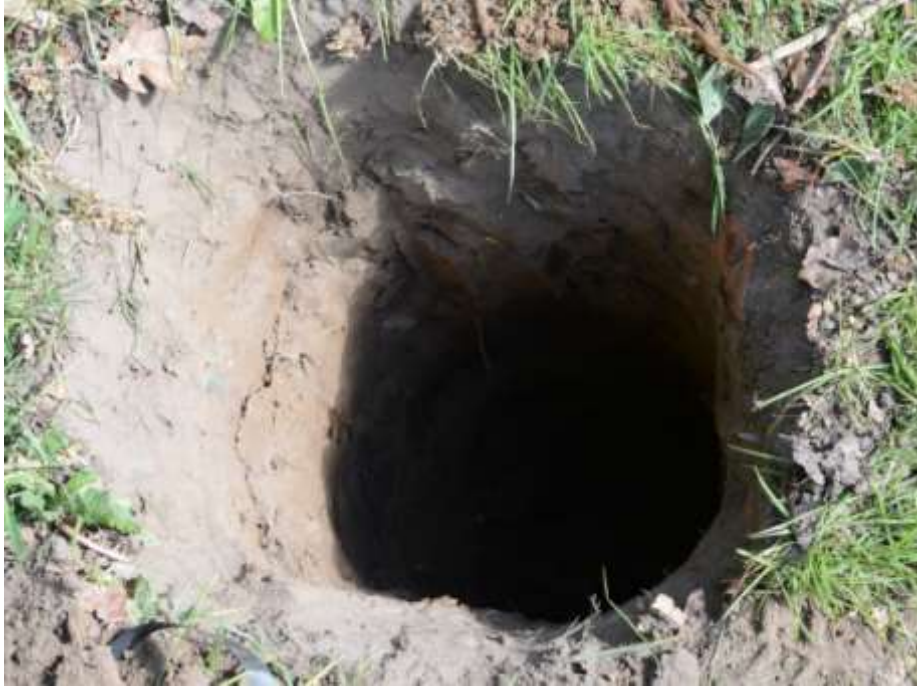
Figure 19: Gate Post Hole 1, facing NW
