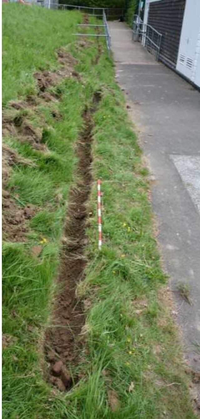
Figure 14: View of cable trench facing NE, 1m scale
