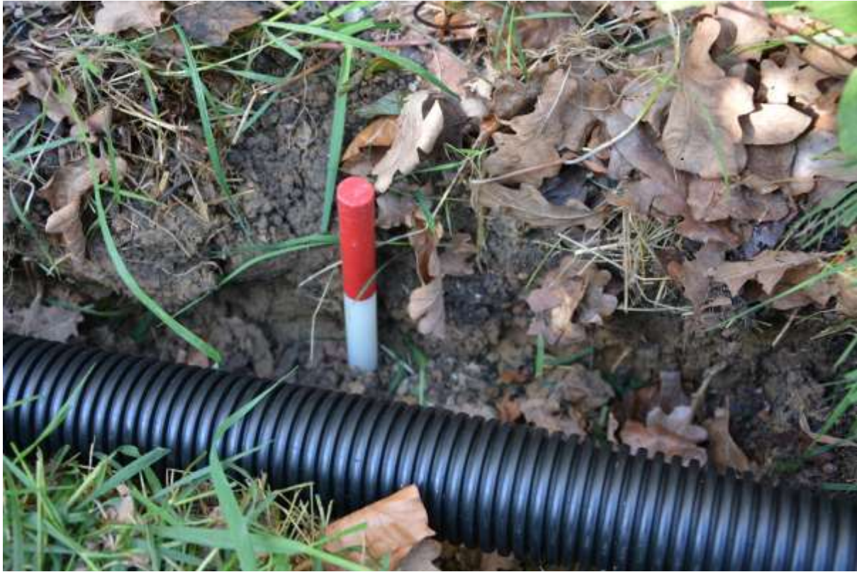
Figure 18: Section of cable trench behind hutted classroom facing SW, 0.2m scale
