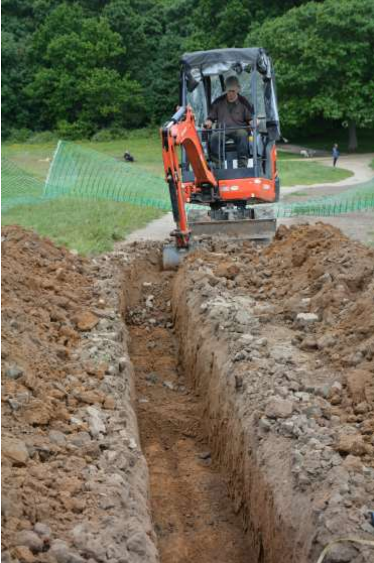
Fig.15: Working shot of Trench 4, facing NNW
