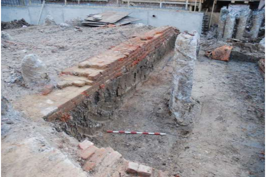
Figure 13: Wall [58], north face. Another brick surface, S[73] can be seen in the foreground. Facing WSW. Scale 1m.
