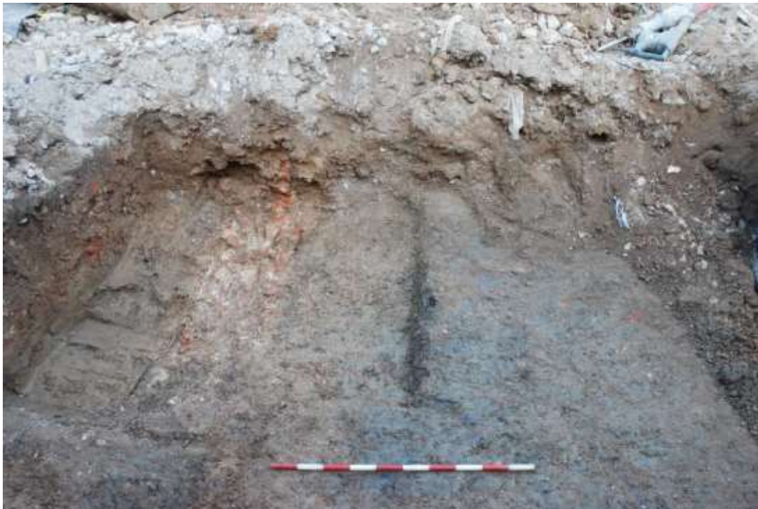
Figure 53: Completed ramp trench, showing modern construction debris overlying stained clay. The drain feature can be seen to the left of frame. Facing E. Scale 1m.
