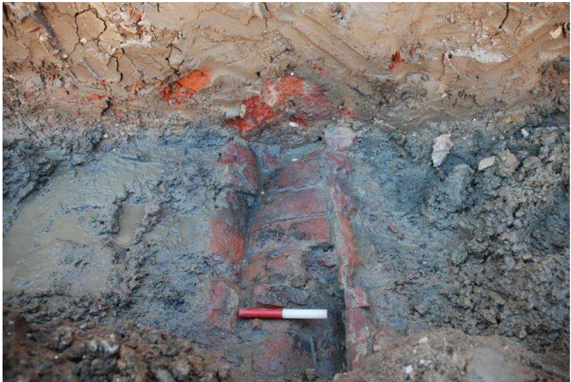
Figure 25: Base of culvert [22] as seen at the western limit of excavation, with the remnants of the arch seen in section. Facing W. Scale 0.2m.
