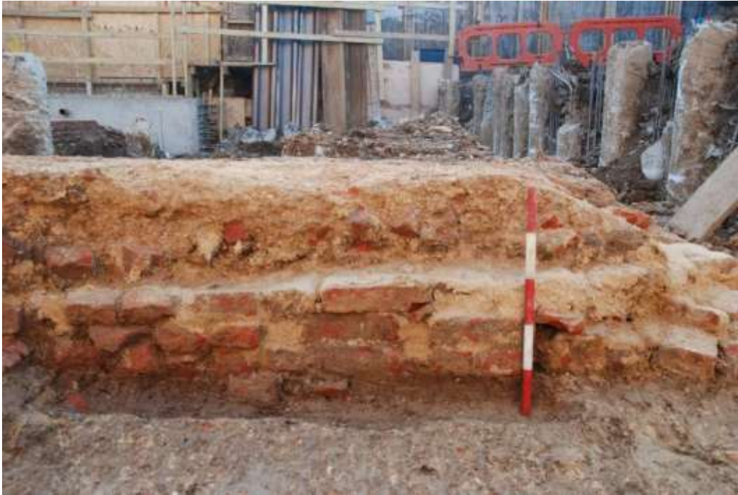
Figure 35: Northern end of wall W[53] showing three courses of surviving brickwork below demolition mortar and rubble. Facing W. Scale 0.5m.
