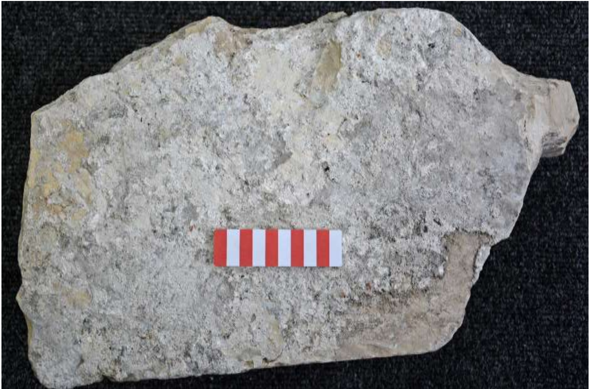
Figure 35: (A) – top of stone, showing remnants of mortar used in bonding stone into sewer, [50] construction. Scale 0.1m
