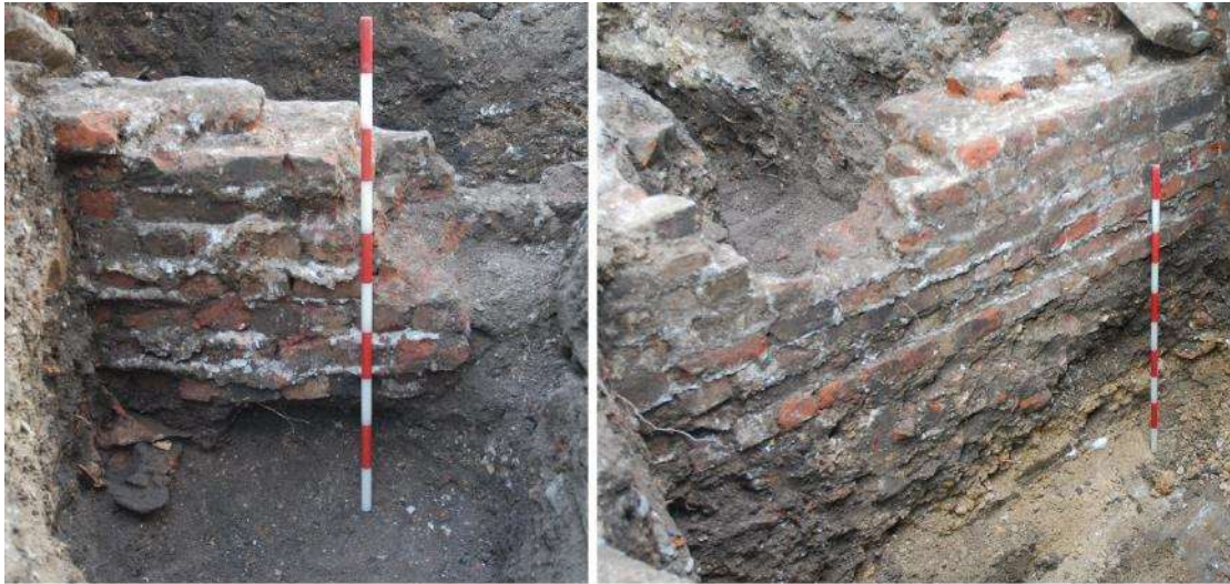
Figure 15: Wall [82] showing E (left) and W (right) sides. Note difference in bond. Scale 1m
