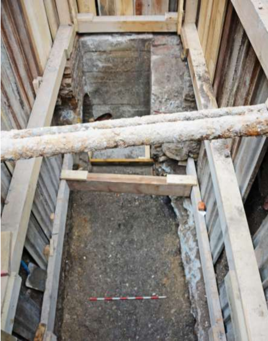
Figure 4: Base of drop shaft looking N. Scale 1m
