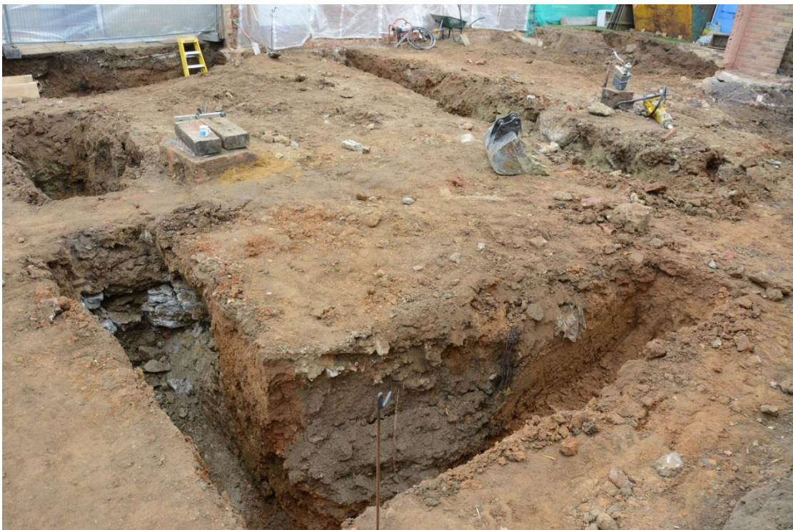
Fig.15: Strip footings for the proposed development, facing SW
