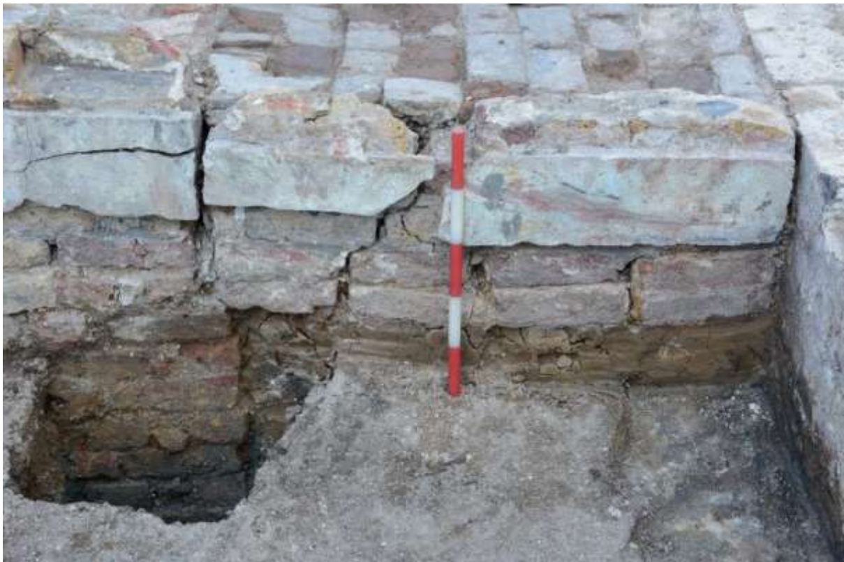
Figure 55: Change in foundation levels between [40] (left) and [39] (right). Note render on courses 2 and 3, and lack on secure bonding to wall [24] (far right) and [40]. Looking NE. Scale 0.5m
