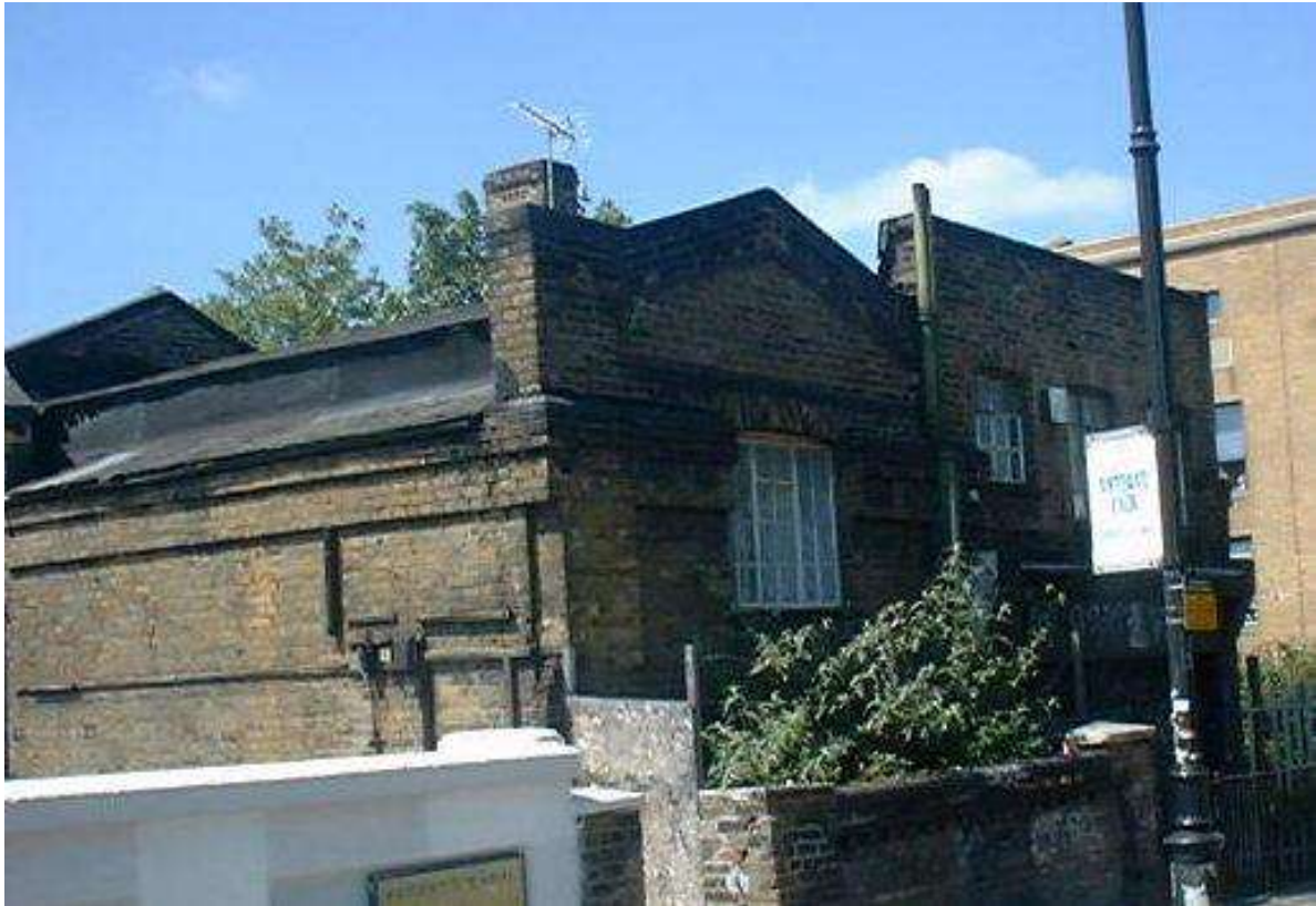
Figure 29: View of the steam pumping station, Kentish Town lock. Looking NW. (2000)
