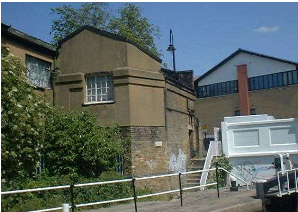
Figure 30: View of the steam pumping house, Kentish Town lock. Looking NE (2000)
