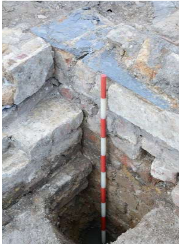
Figure 57: Showing insecure bond and foundation difference between [30] (left) and [40]. Note course of slates as damp proofing in [40]. Looking N. Scale 1m.
