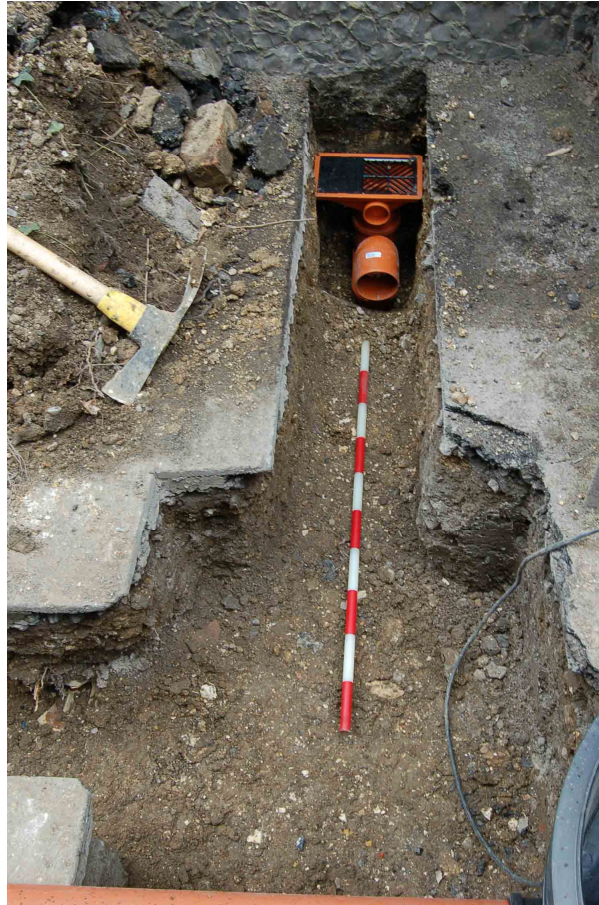
Fig 14: North-south section of Trench 6, looking south.
