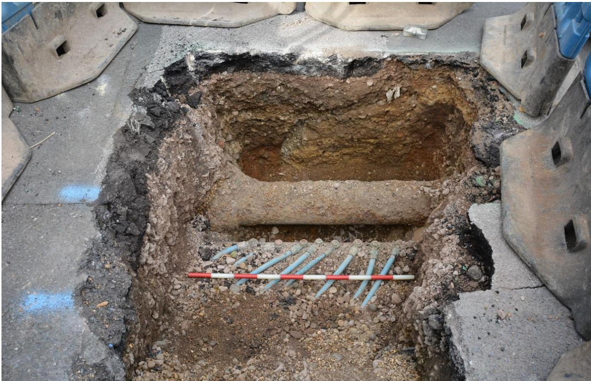
Figure 10: Trench 3, located within the existing carriageway. Facing W. Scale 1m.
