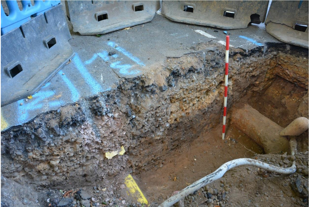
Figure 7: North facing section of Trench 1, showing the gravels and light sandy soil below the road surface. Orange sand can be seen towards the base of the section, with service cut [7] to the left of frame. Facing SW. Scale 1m.
