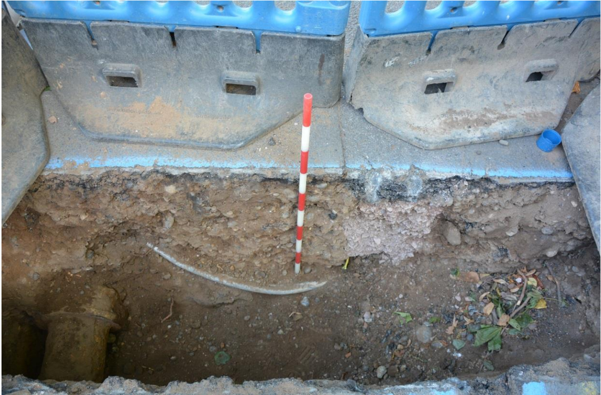
Figure 9: South facing section of Trench 2, showing made ground and services below the road surface. Facing N. Scale 1m.
