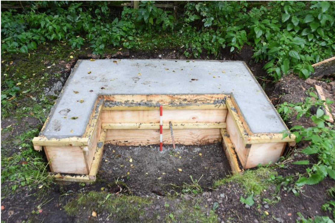
Figure 7: The substation base. Looking N. Scale 0.5m
