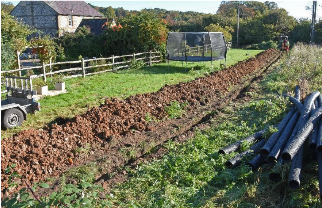
Figure 12: Overview of E-W trench. Looking NE. No scale
