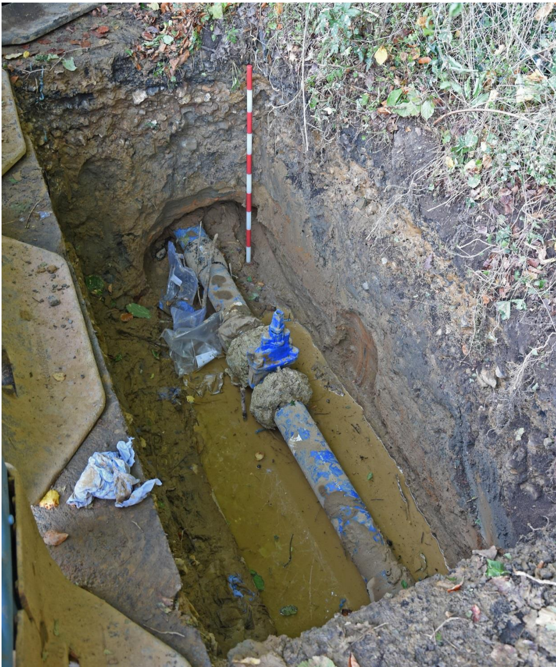
Figure 10: Pit 3. Looking E. Scale 1m.
