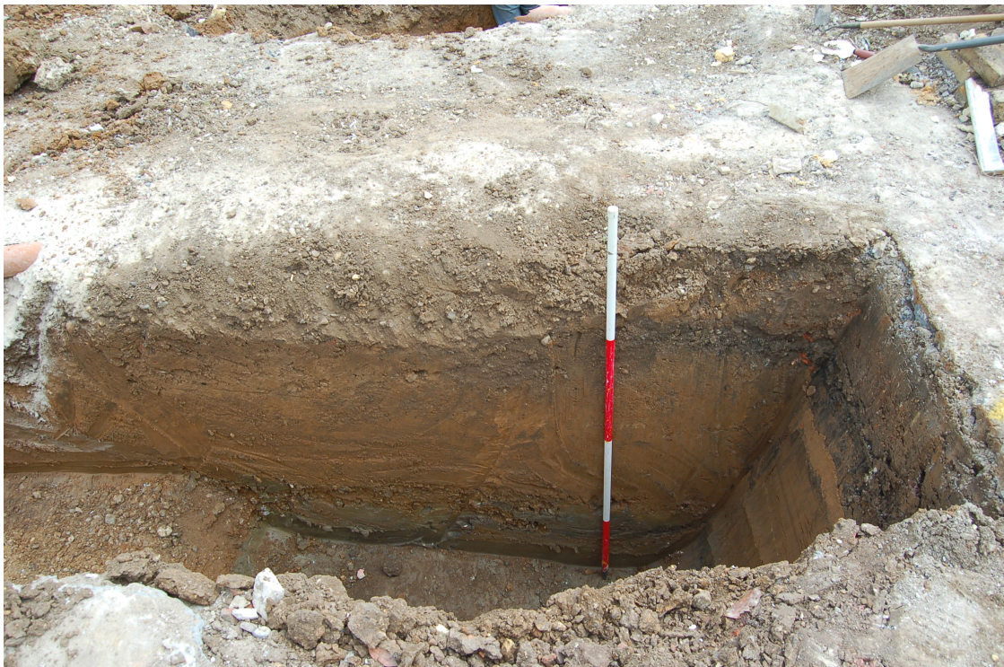
Fig 8 View of Trench 2 looking towards the northwestern section (2m Scale). The depths of concrete and firm alluvial clay can be clearly seen. The gravel lens is just evident above the last red block of the scale and the blue clay can be seen appearing below this point.
