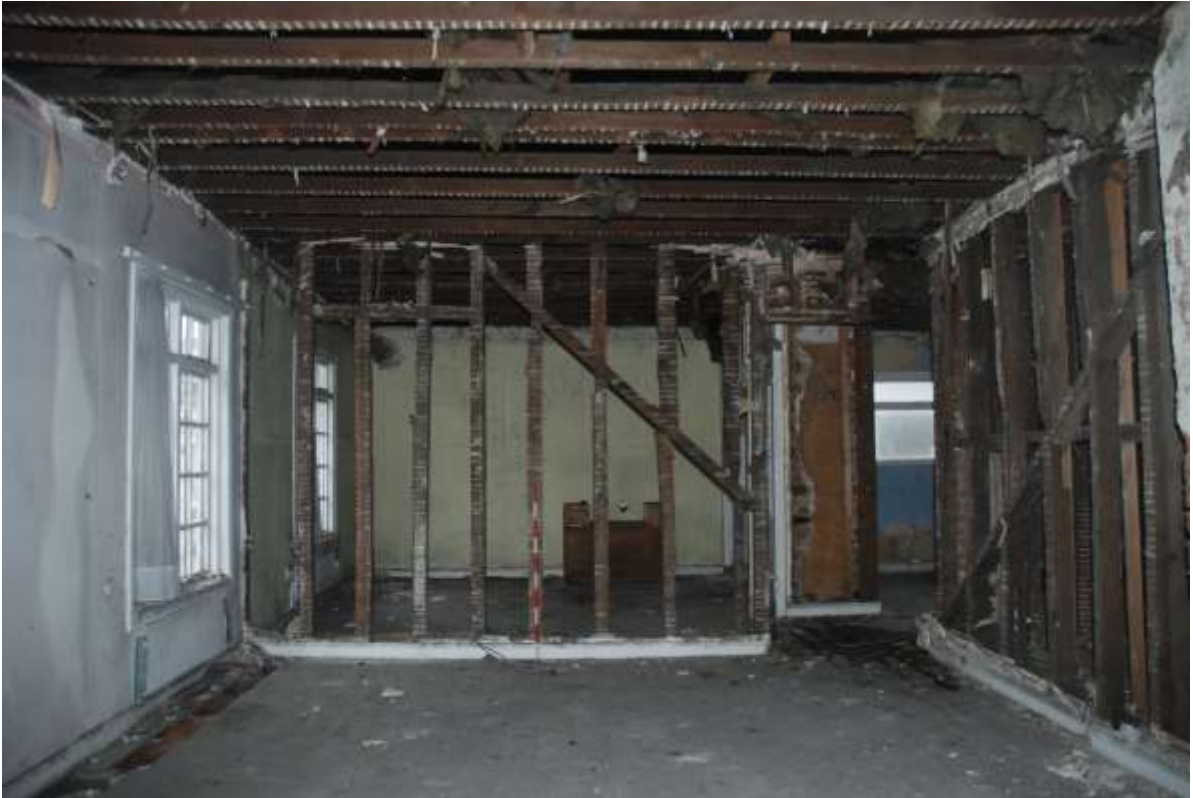
Fig.85: Room F4 facing N, 1m scale
