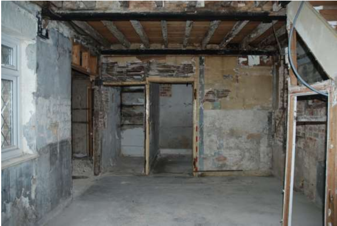
Fig.50: Room G4 facing W, 1m scale. Room G2 through door by scale, room G3 to left of this
