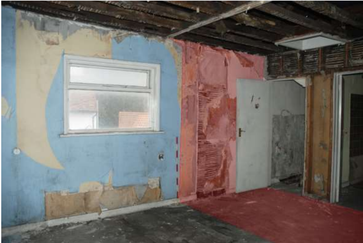
Fig.73: Room F1, and hallway, (shaded red), facing NE
