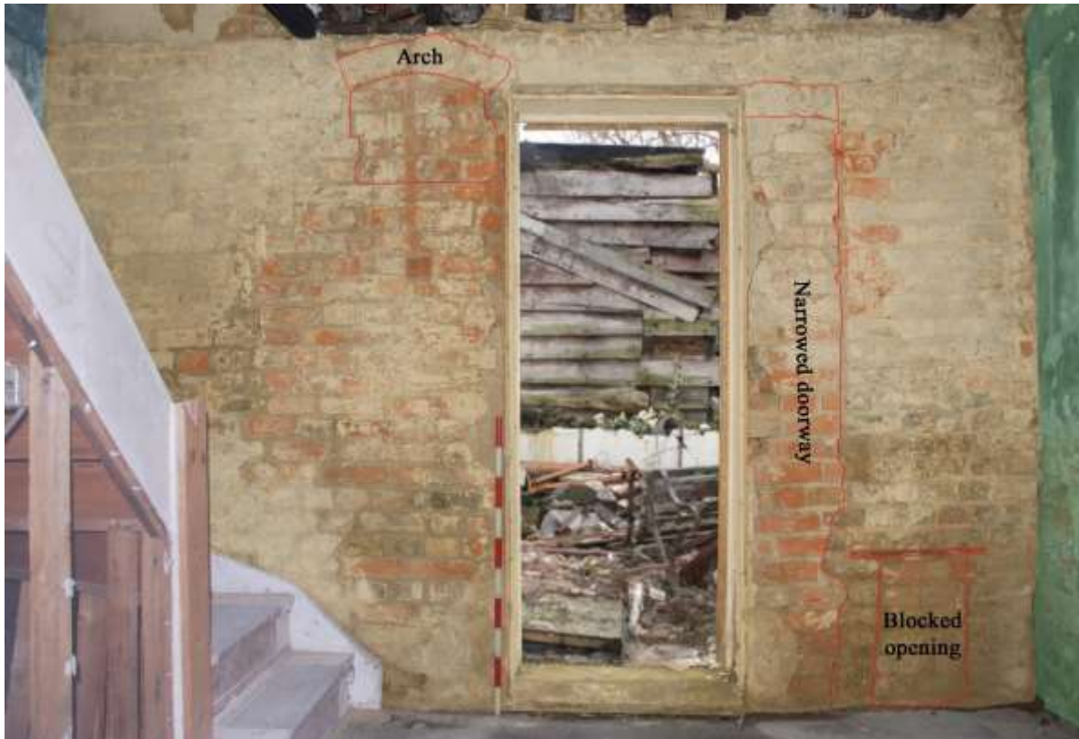
Fig.54: Eastern wall of room G4 with external door, 1m scale. Green is earliest phase, orange second, purple third. Blocked up elements outlined in red
