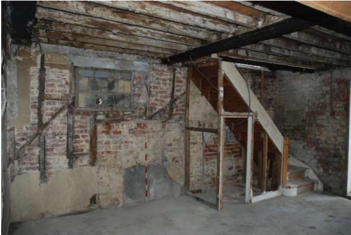
Fig.52: The northern (external) wall of room G4 facing NE, 1m scale
