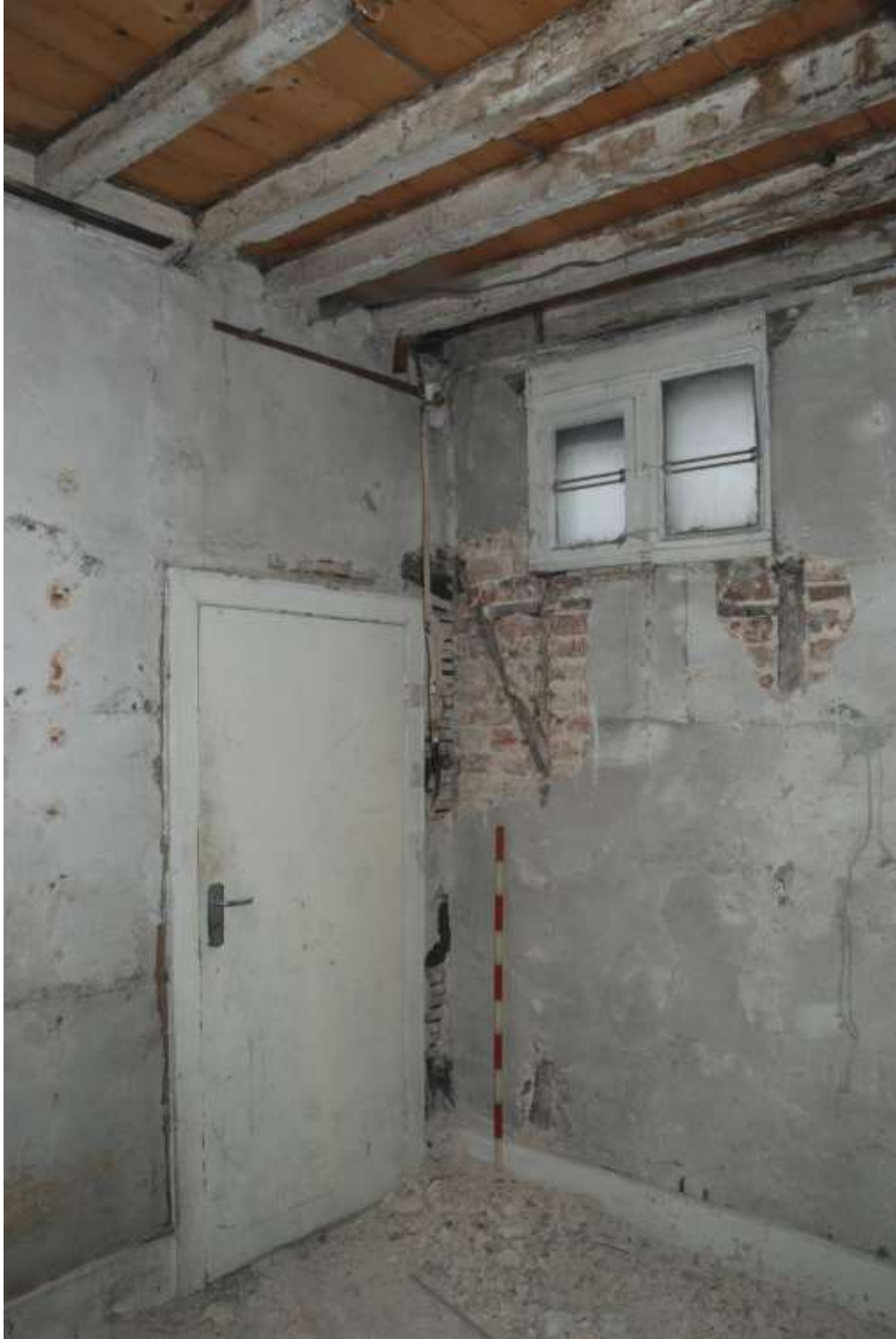
Fig.40: Room G2 facing NW, 1m scale
