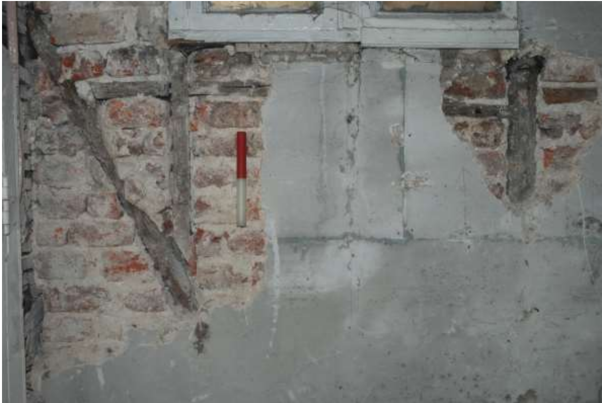
Fig.43: Detail of north wall showing timber framework, brick infill and plaster finish. 0.20m scale
