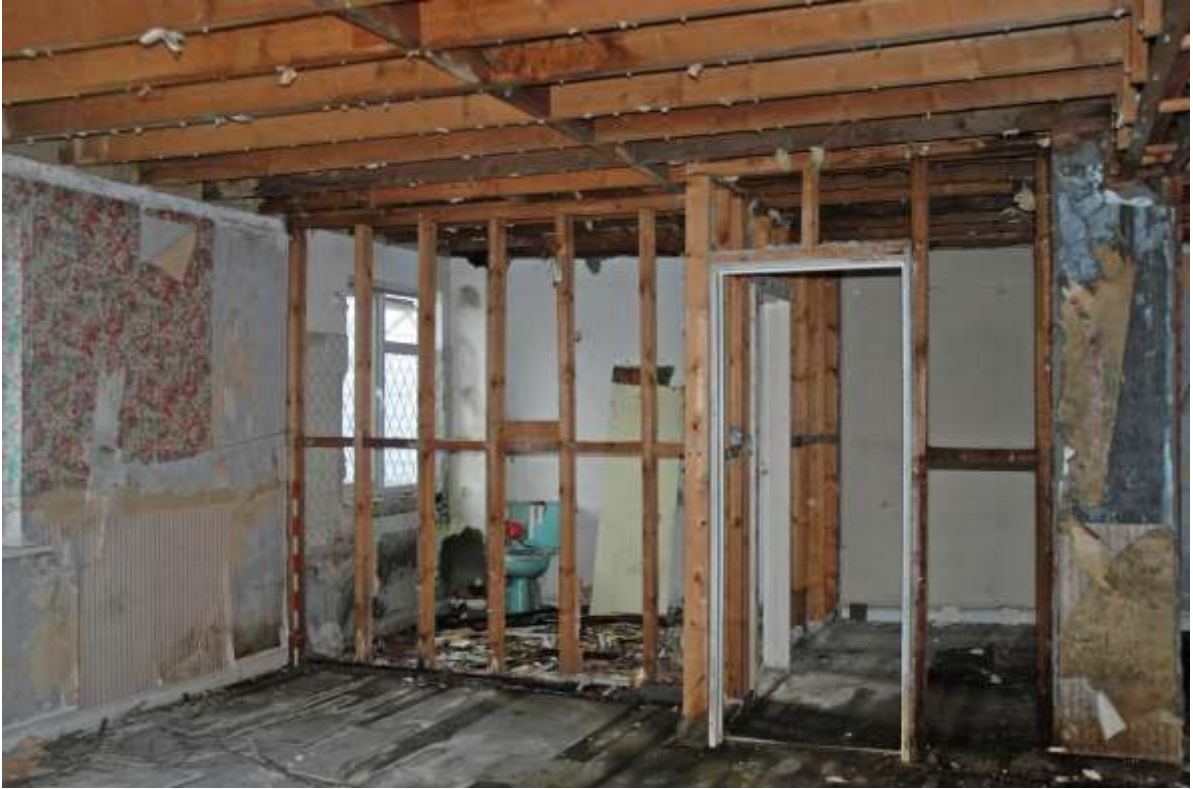
Fig.91: Room F5, facing SE, 1m scale. Door to F6 and toilet in the background
