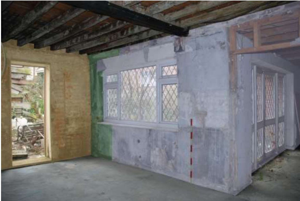
Fig.57: Room G4 facing SE, 1m scale. Earliest phase in green, second in orange, third in purple
