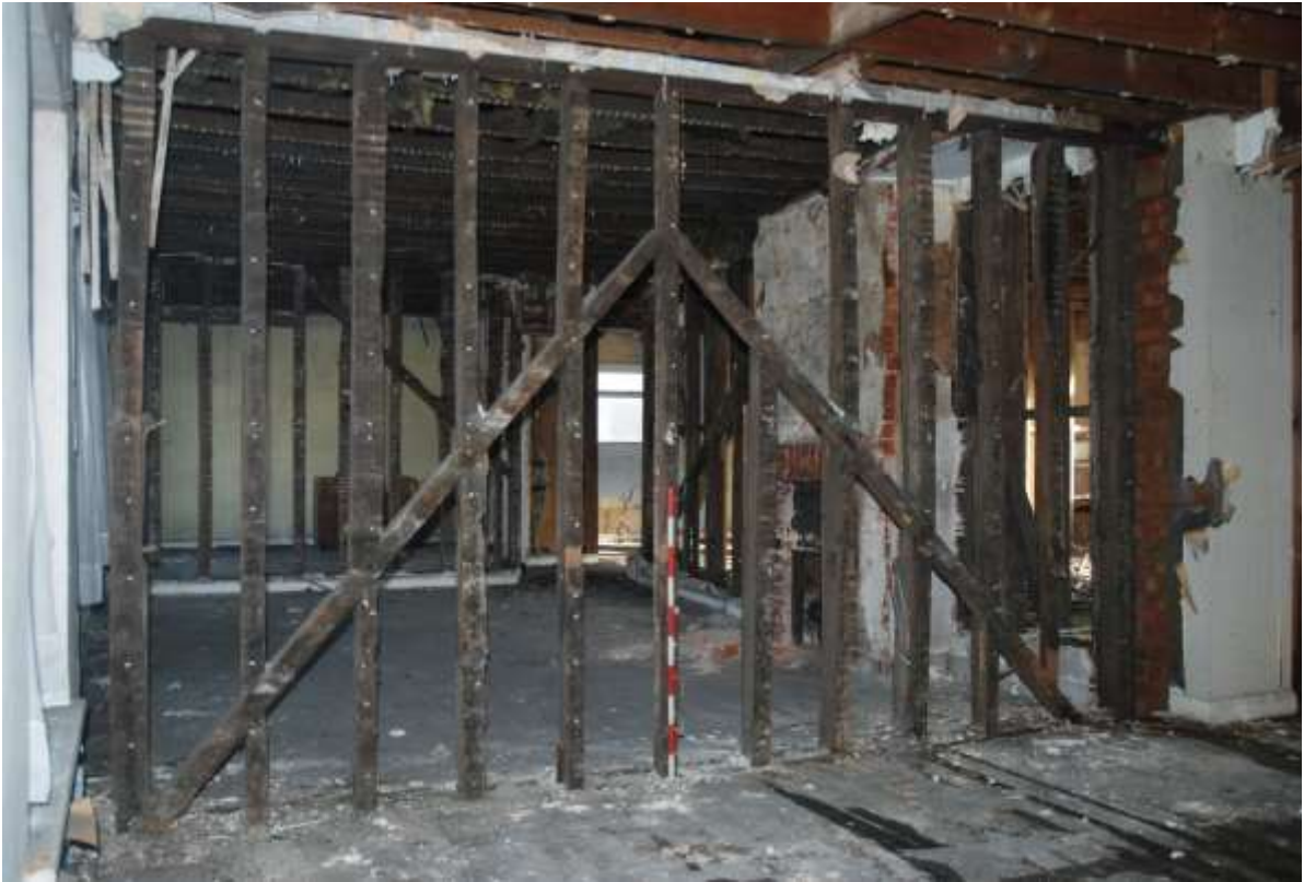
Fig.97: Room F6, facing, NE, 1m scale
