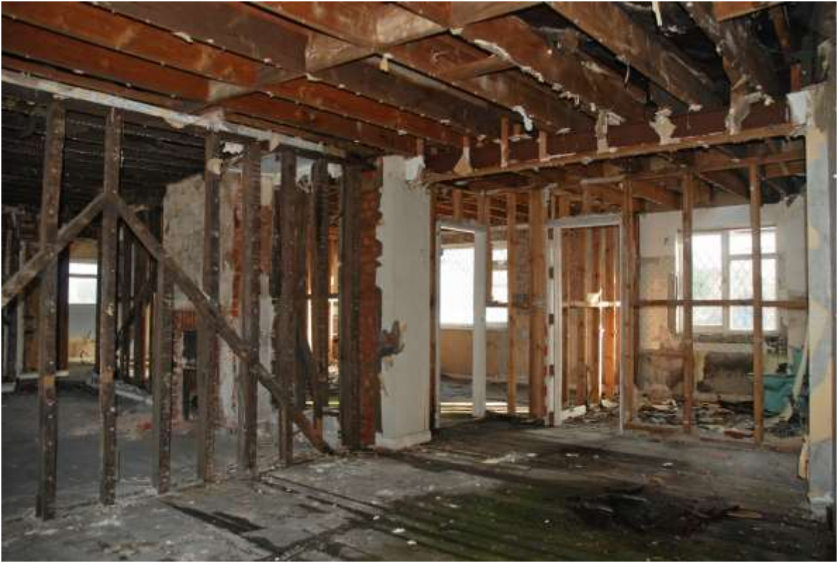
Fig.98: Room F6, facing NE, 1m scale
