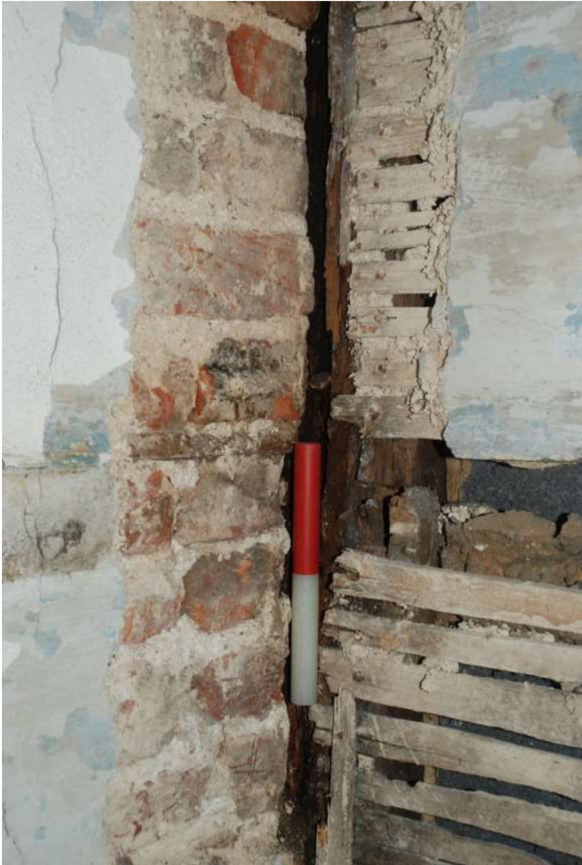
Fig.48: Detail of the SW corner of G3 facing SW, 0.20m scale. Note the brickwork abutting the lath and plaster on the western wall
