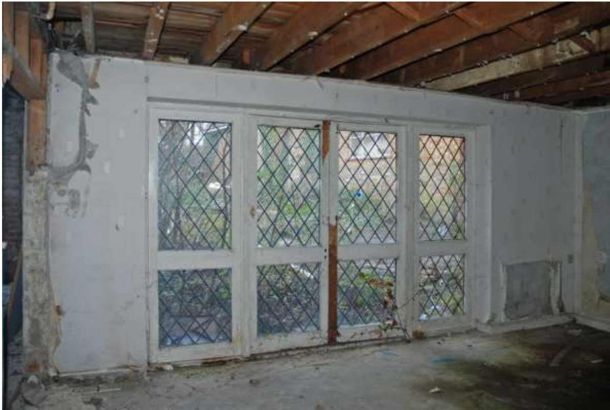
Fig.63: East wall of room G6, facing SE, showing the French doors
