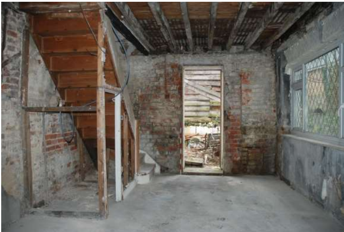
Fig.51: Room G4 facing E, 1m scale
