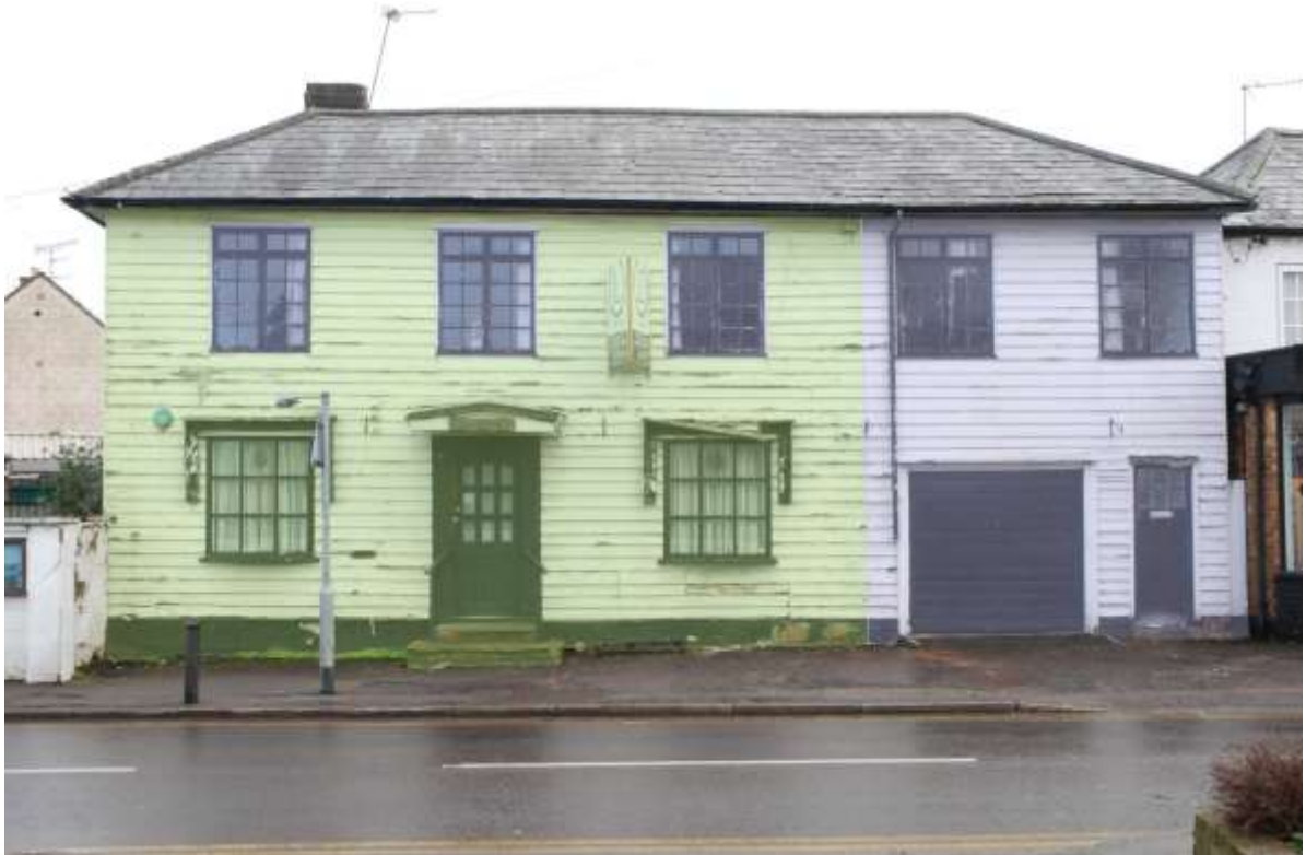
Fig.12: Western frontage facing E, showing the original core, (green), and the modern extension to the south, (purple)
