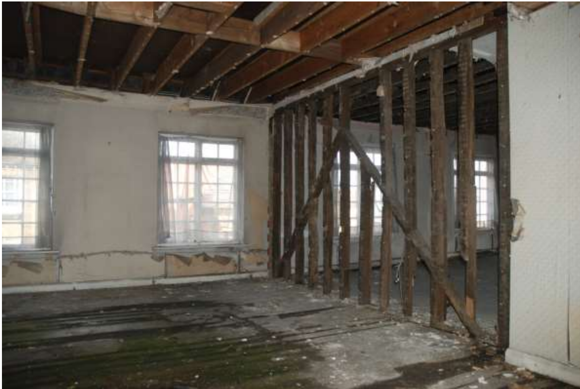
Fig.96: Room F7, facing WNW, 1m scale
