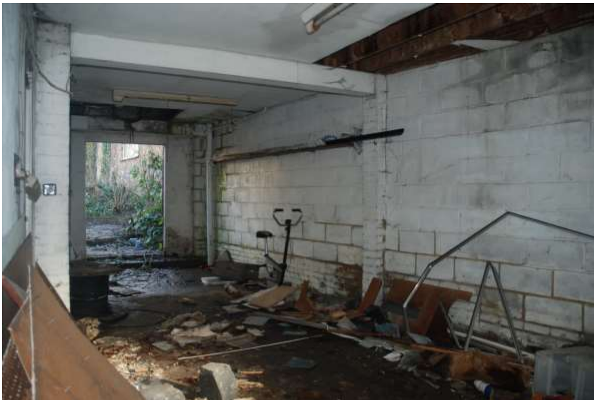
Fig.68: Garage facing SE, note the breeze-block construction
