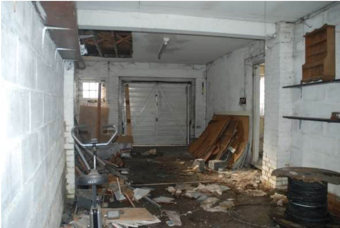
Fig.66: Garage space facing NW towards frontage
