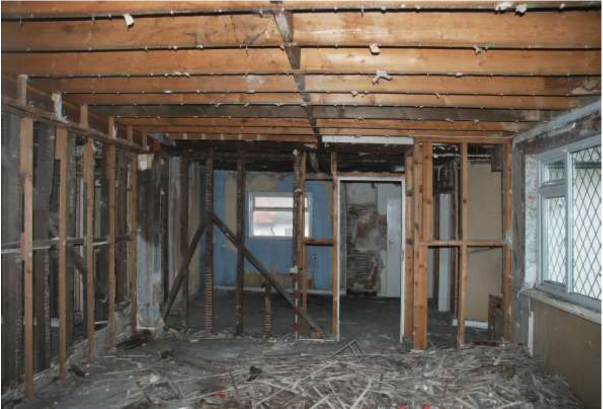
Fig.92: Room F5, facing N, 1m scale
