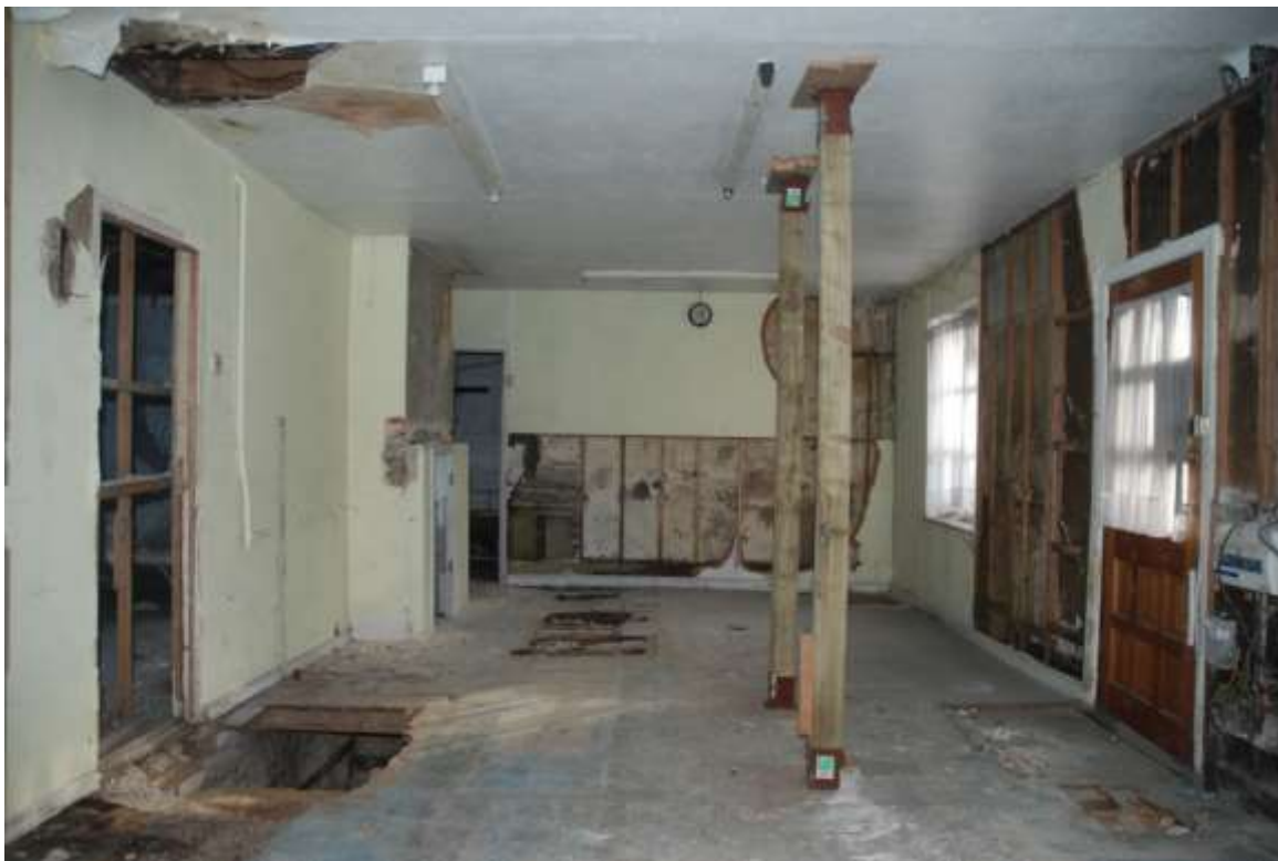
Fig.27: Room G1 facing S, eastern cellar walls just visible in left foreground. 'Scars' of former hallway walls also visible as slightly raised lines in the ceiling
