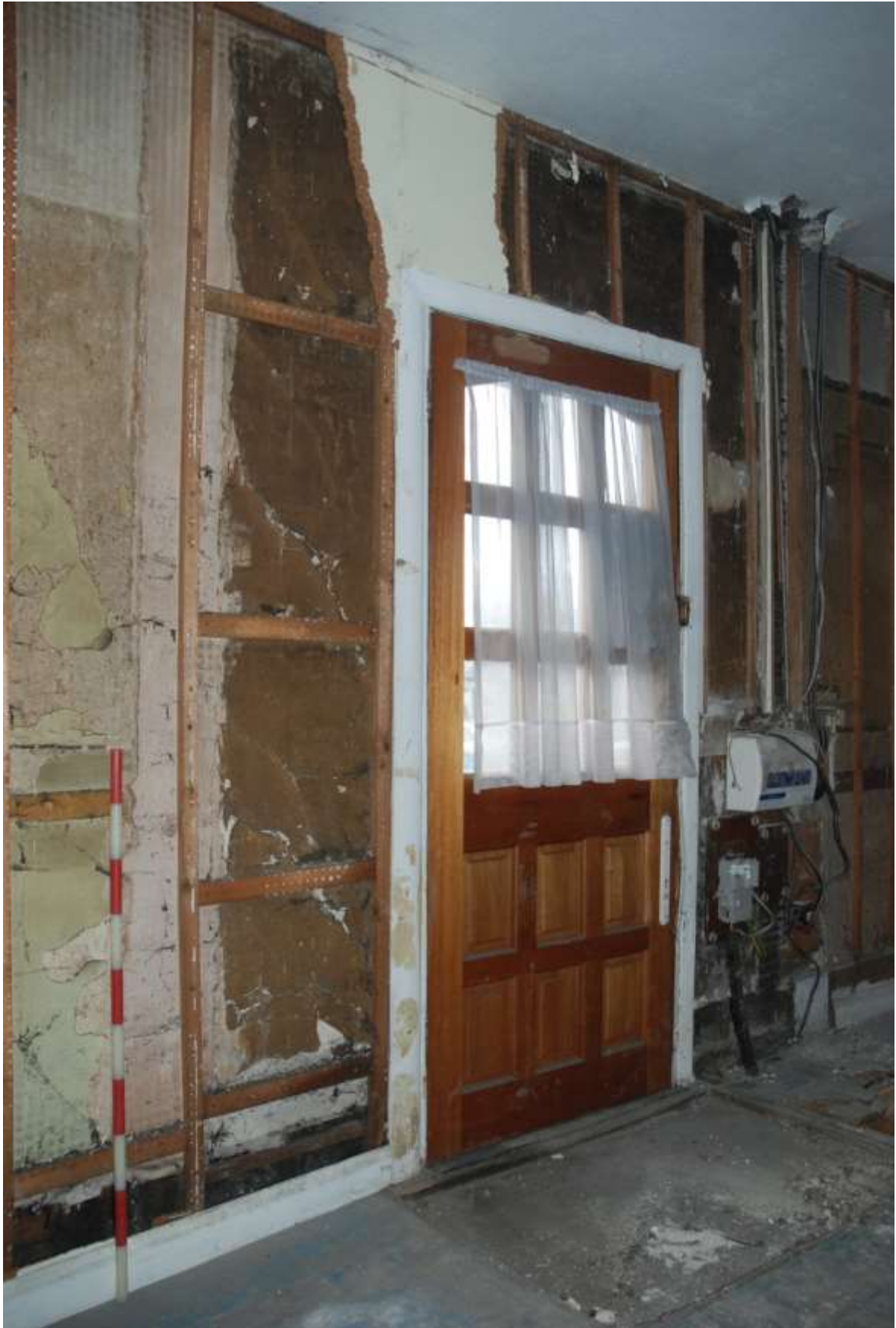
Fig.31: Front door in west wall, Room G1, facing NW, 1m scale. Note the 'scar' of the former southern wall of the hallway in bare plasterwork.
