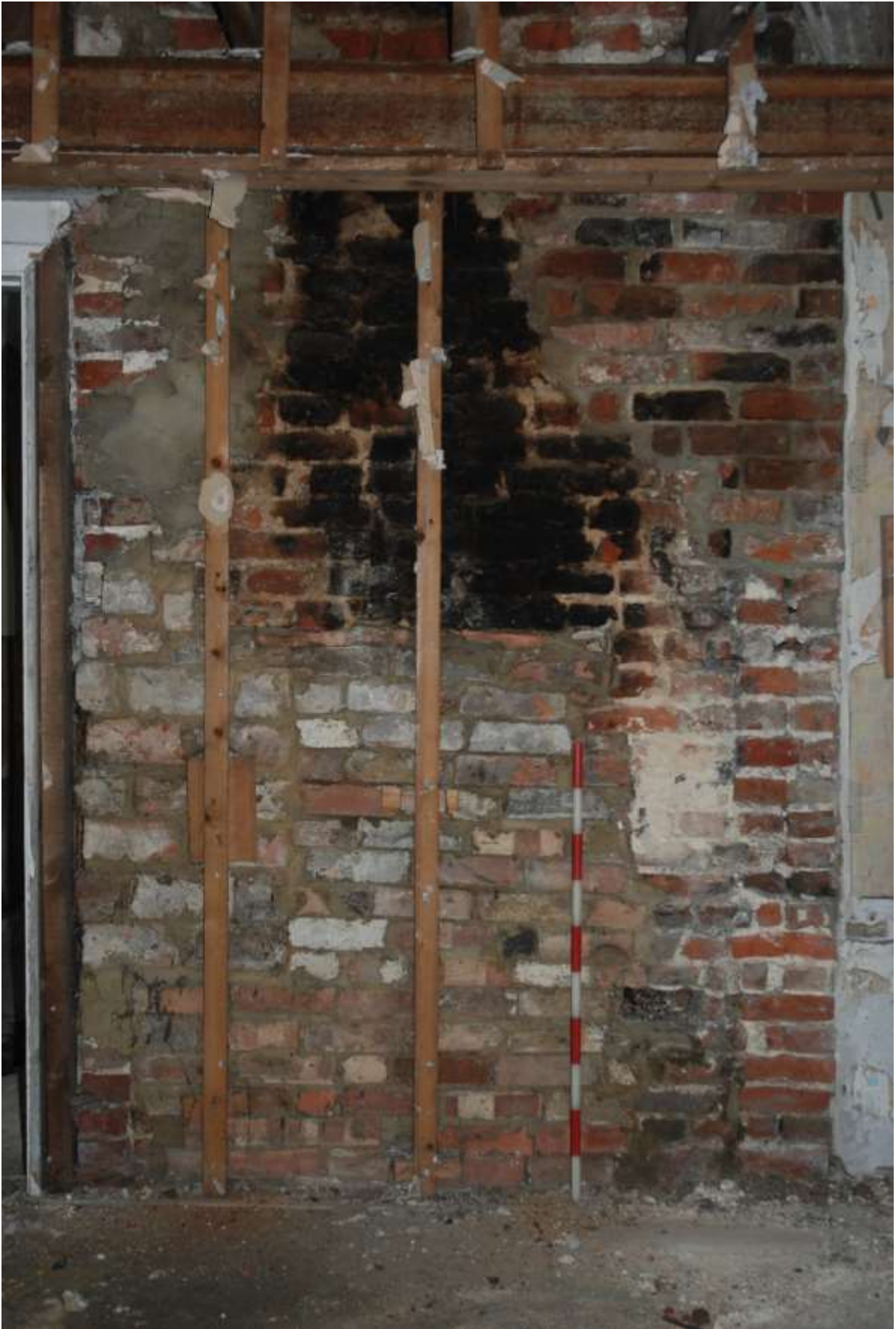
Fig.64: Detail of former fireplace, facing W, 1m scale
