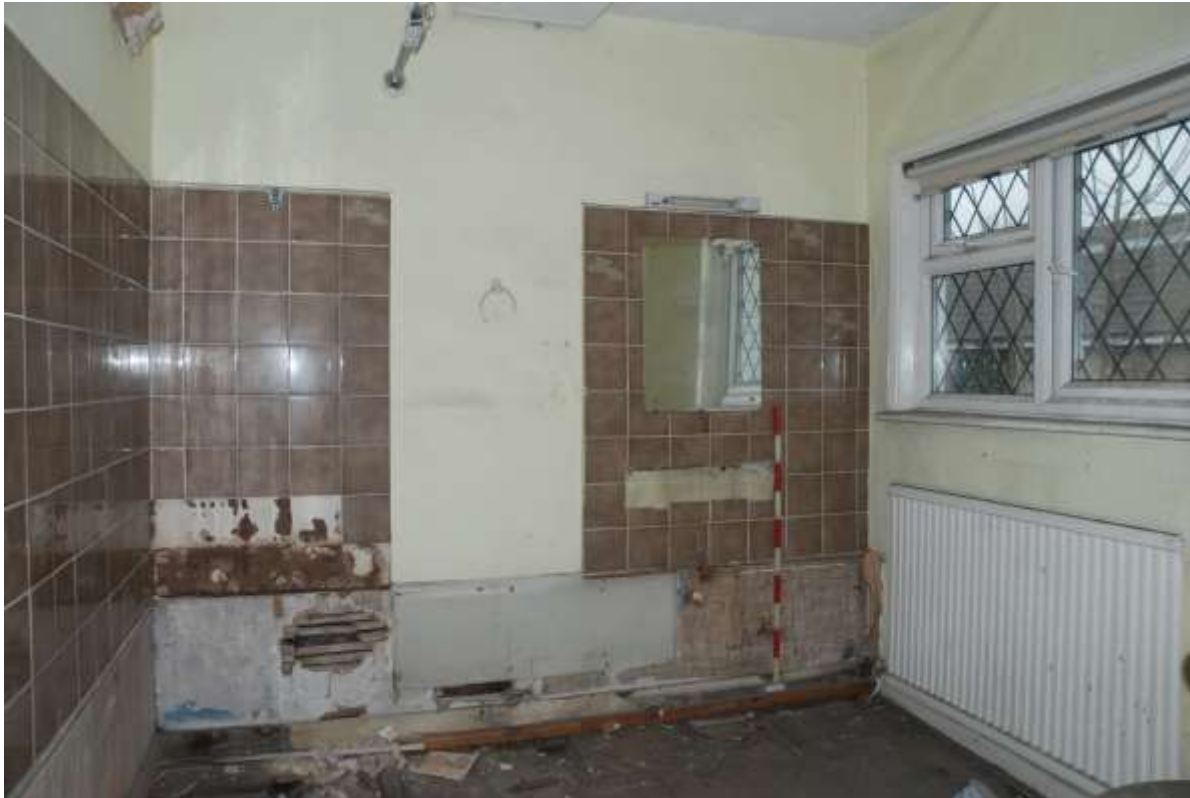
Fig.76: Room F2, bathroom, facing ESE, 1m scale
