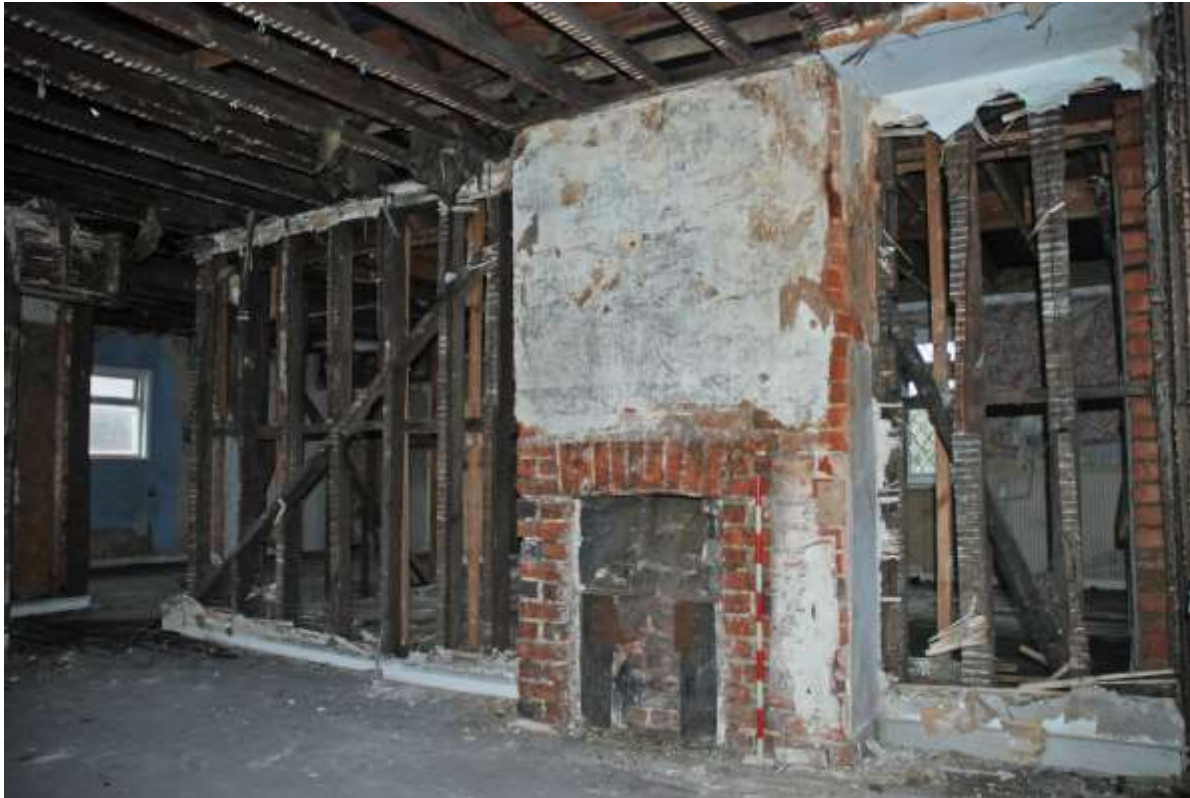
Fig.87: Room F4, facing NE, 1m scale, southern chimney stack
