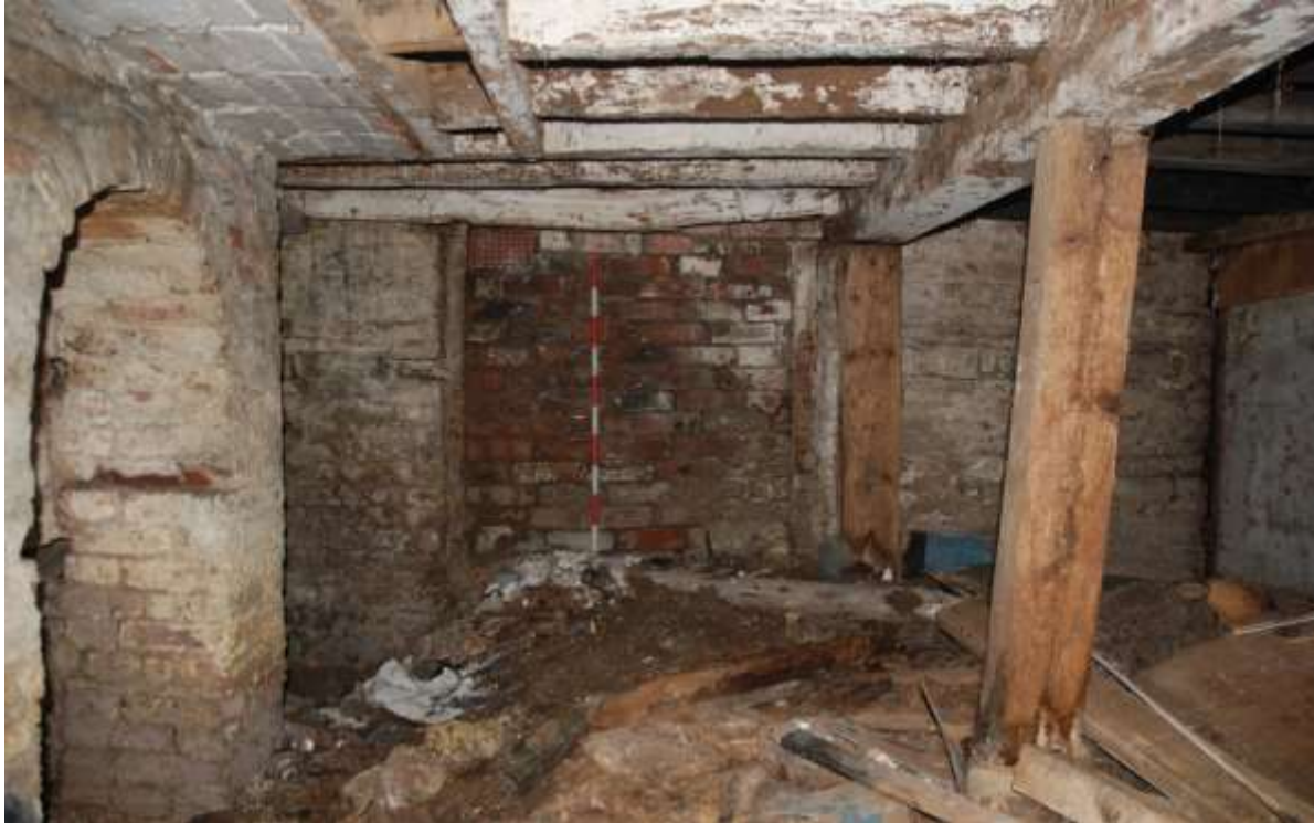
Fig.22: South wall facing S, showing the brick-up access point. 1m scale
