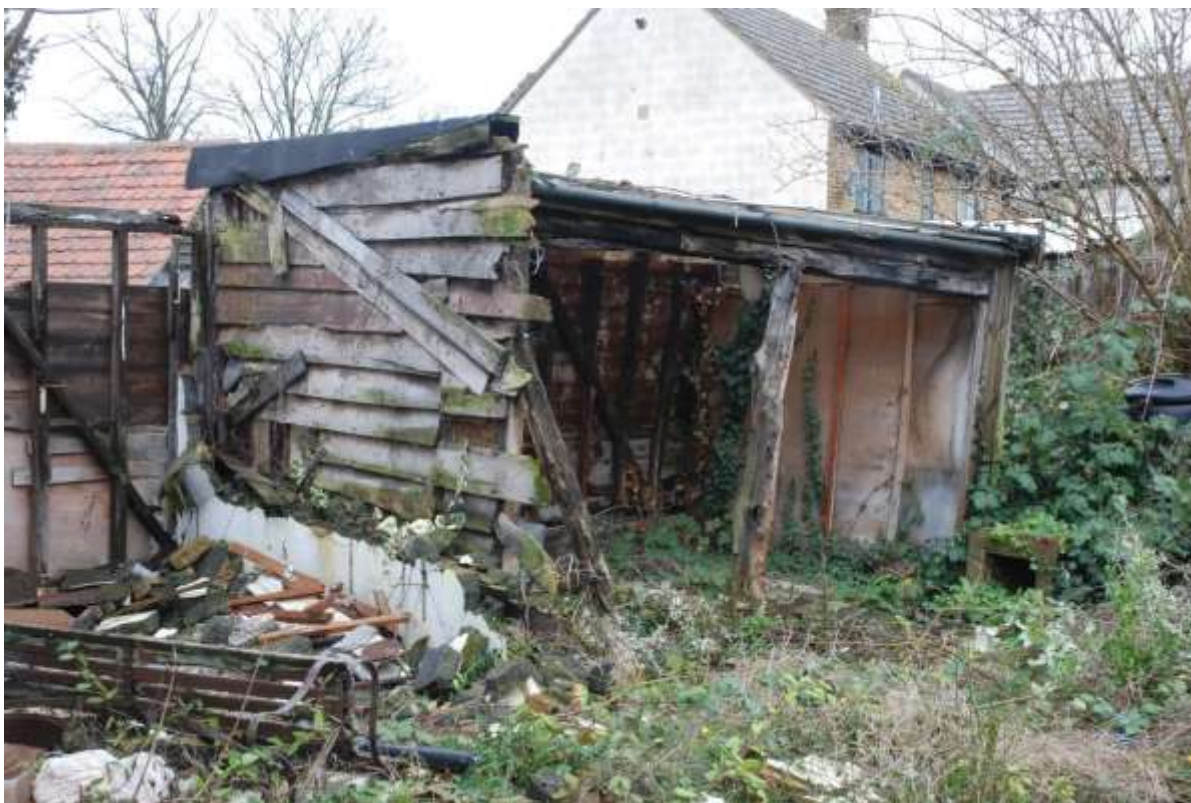
Fig.106: Shed facing NE
