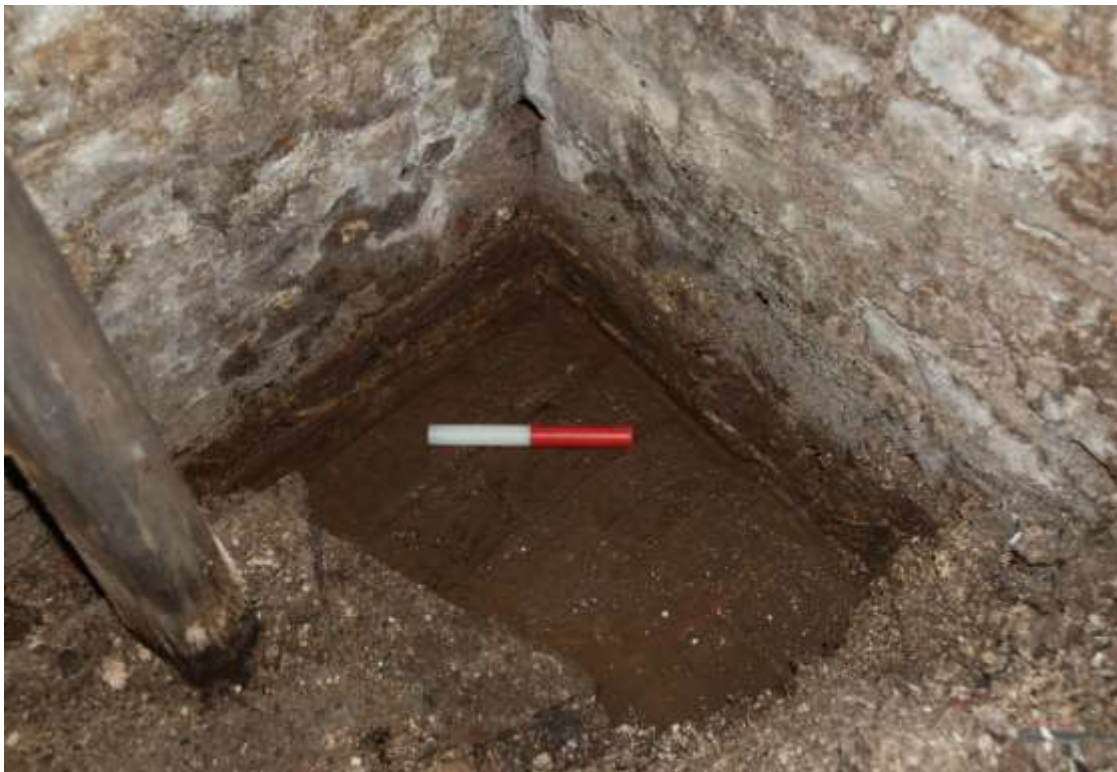
Fig.20: Exposed brick floor in SE corner, 0.20m scale
