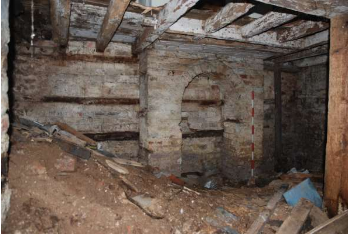
Fig.21: East wall of the cellar, facing SE, 1m scale. Note the brick support for the southern fireplace in room G1 above
