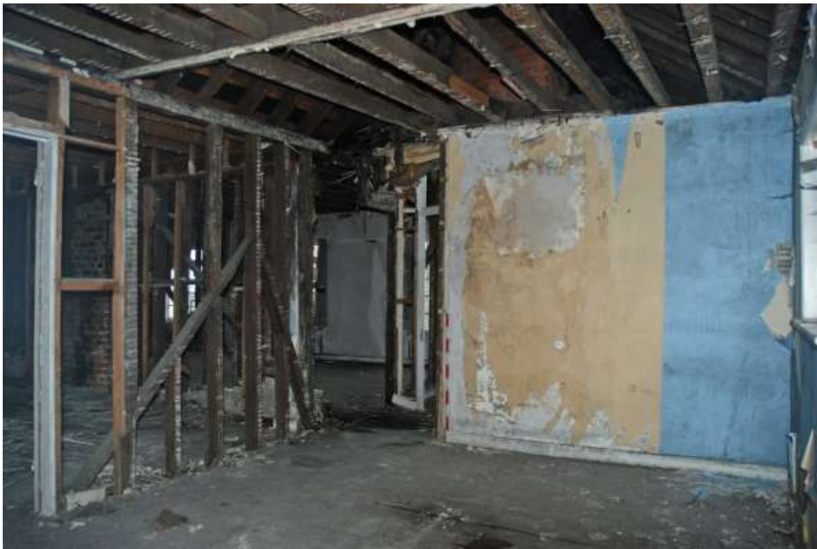
Fig.74: Room F1 facing SW, 1m scale
