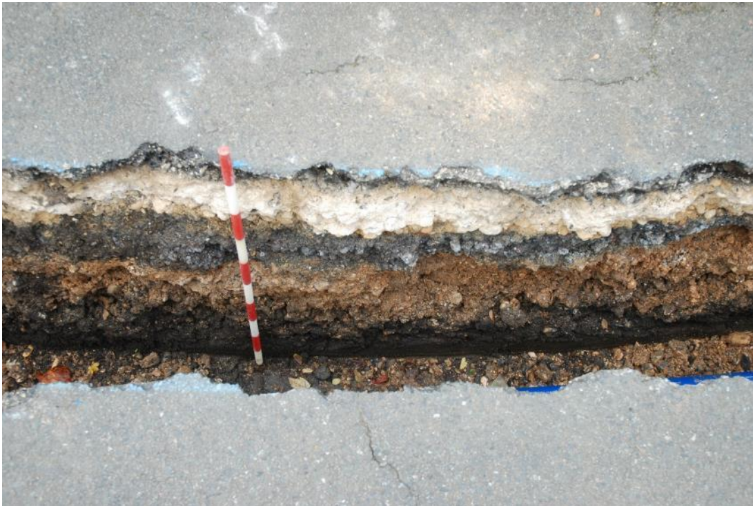
Figure 9: Darker silty clay (6) seen towards the trench base. Facing NW. Scale 1m.
