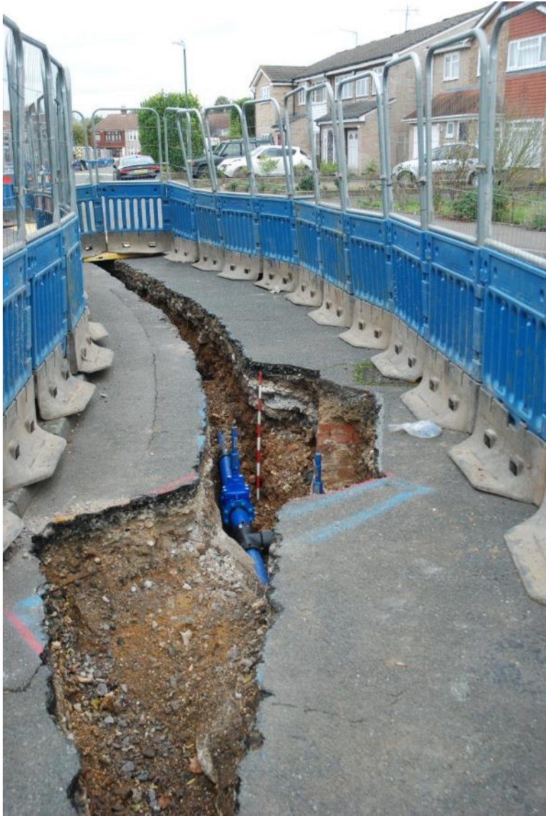
Figure 8: Trench 8. Road make up and gravel layers, (5) and (4). Facing NNE. Scale 1m.
