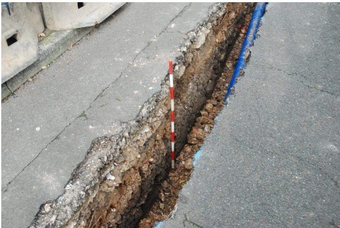
Figure 10: A similar stratigraphy of road make up and gravels overlying a darker, wetter clay was seen throughout Trench 8. Facing NW. Scale 1m.
