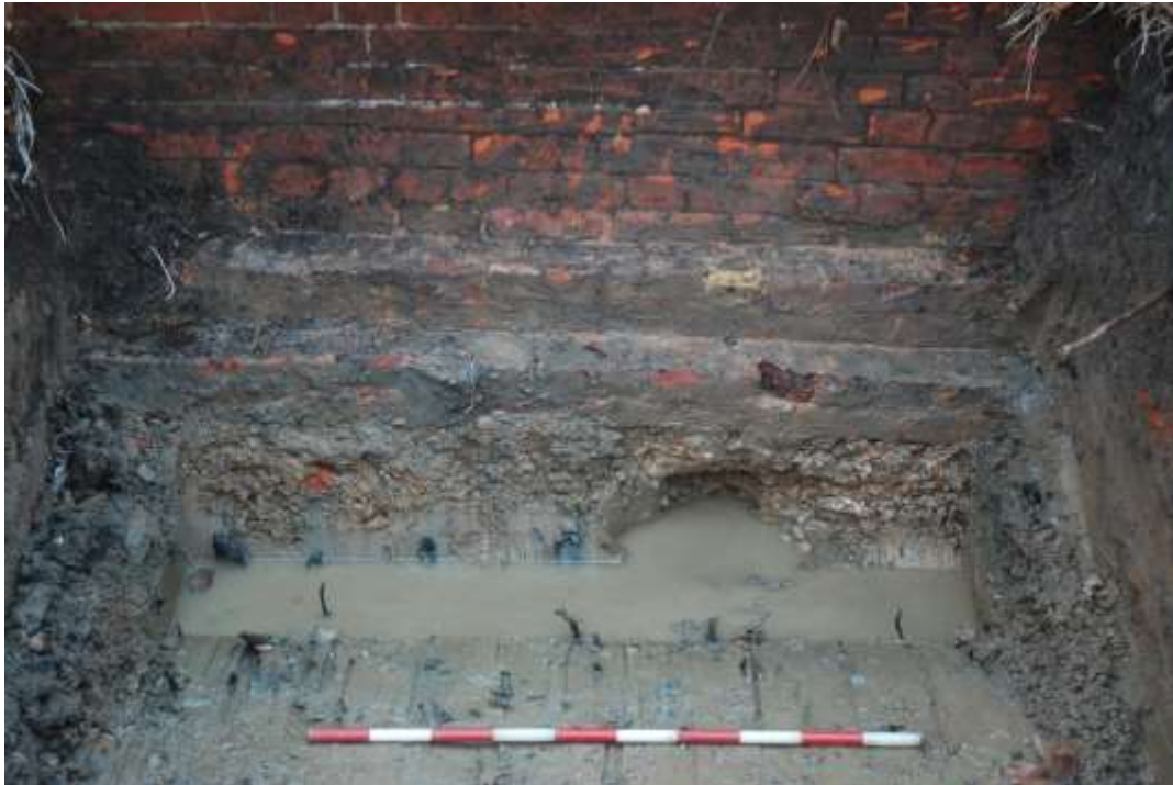
Figure 14: Detail of wall foundation [4] and gravel (5), overlying natural clay (3). Facing SE. Scale 1m.
