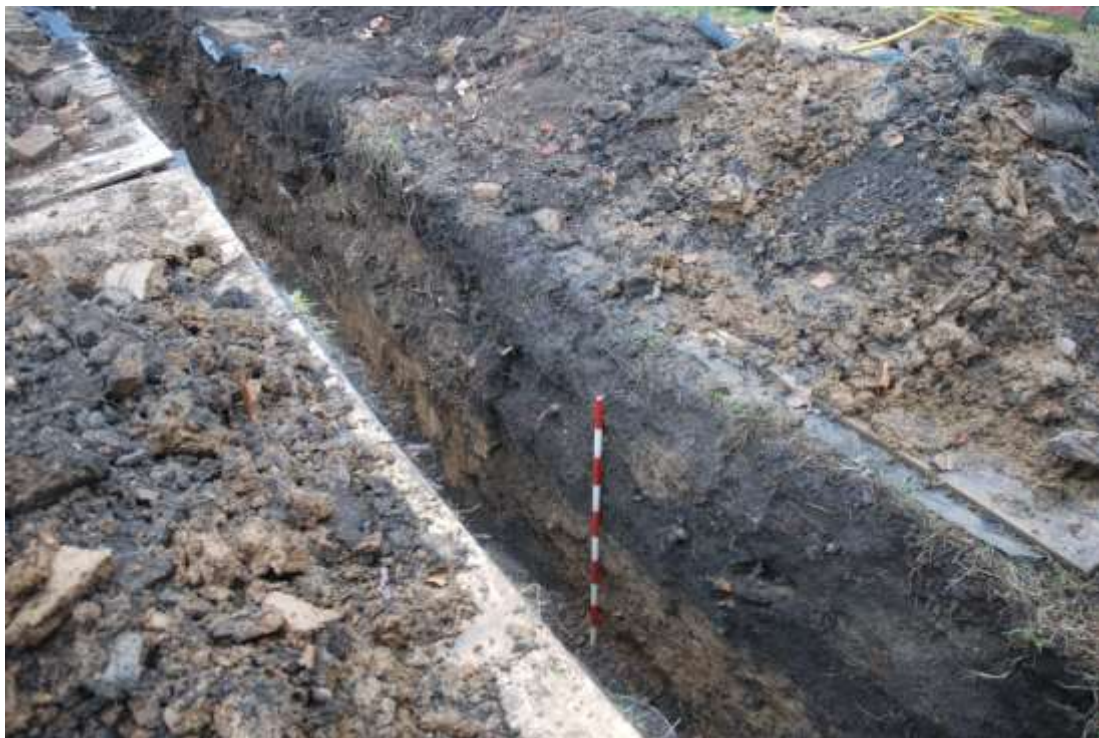
Figure 9: View of TP29 from the northern end, showing topsoil (8) overlying natural clay (11) to the right of the scale, and the beginning of the rubble (10) to the left, with the natural clay sloping downwards towards the canal. Facing approximately SW. Scale 1m.
