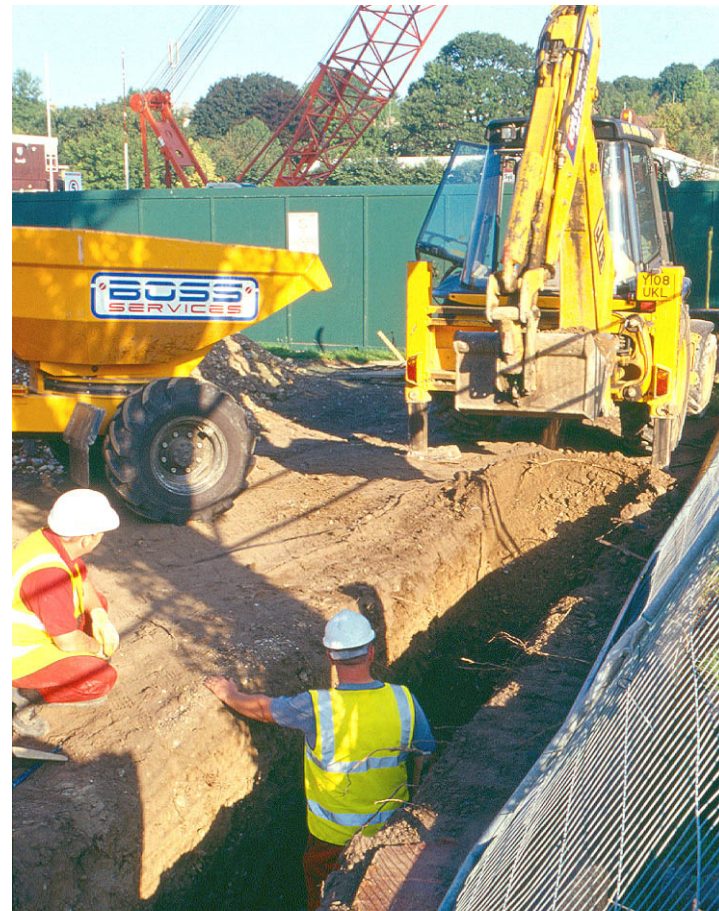
Fig 18 Pipe trench excavation in the playing fields (Area 4 on Figure 15): top left - section just south of the site compound showing the shallow soil horizon and underlying lighter silty (colluvial) deposit, over a former land surface and natural gravel. Bottom left - work in progress. Top & bottom right - views of the fills and overlying deposits in the central and northern parts of the buried stream channel [7] (0.5m scale). The darker waterlaid silt [6] is particularly clear at the base of the lower frame
