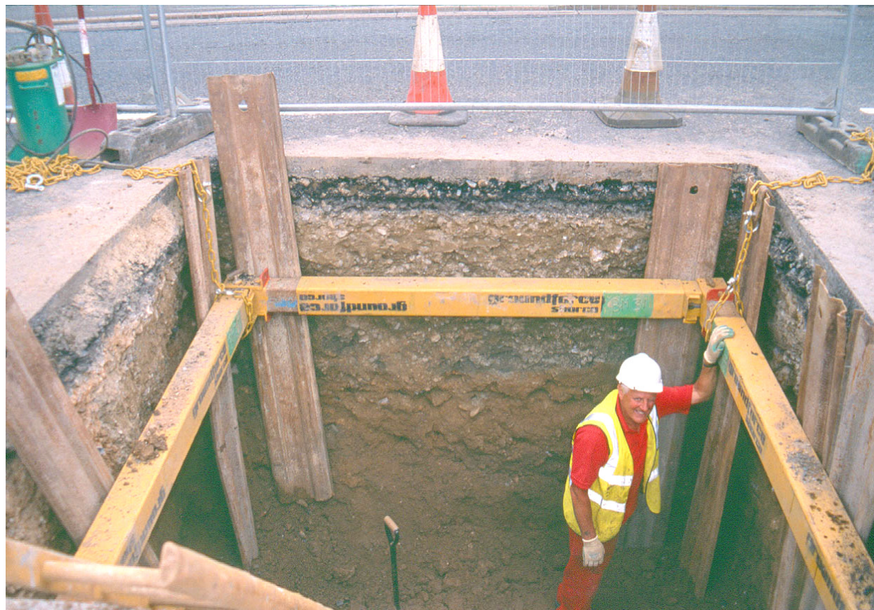
Fig 17 Excavation on Corkscrew Hill (Area 2 on Figure 15): top left – the northern limit of excavation, showing modern road make-up over a clean silty deposit, with natural gravel at a depth of about 1.25m. Bottom left - pit at the southern end of excavation, looking east: the road base overlies c 0.9m of recent made ground, with a remnant buried land surface below and natural gravel at a depth of c 1.35m. Right top & bottom – the main section of pipe trench, general view southeast and detail of the eastern section, both showing recent made ground over disturbed natural gravel (0.5m scale)
