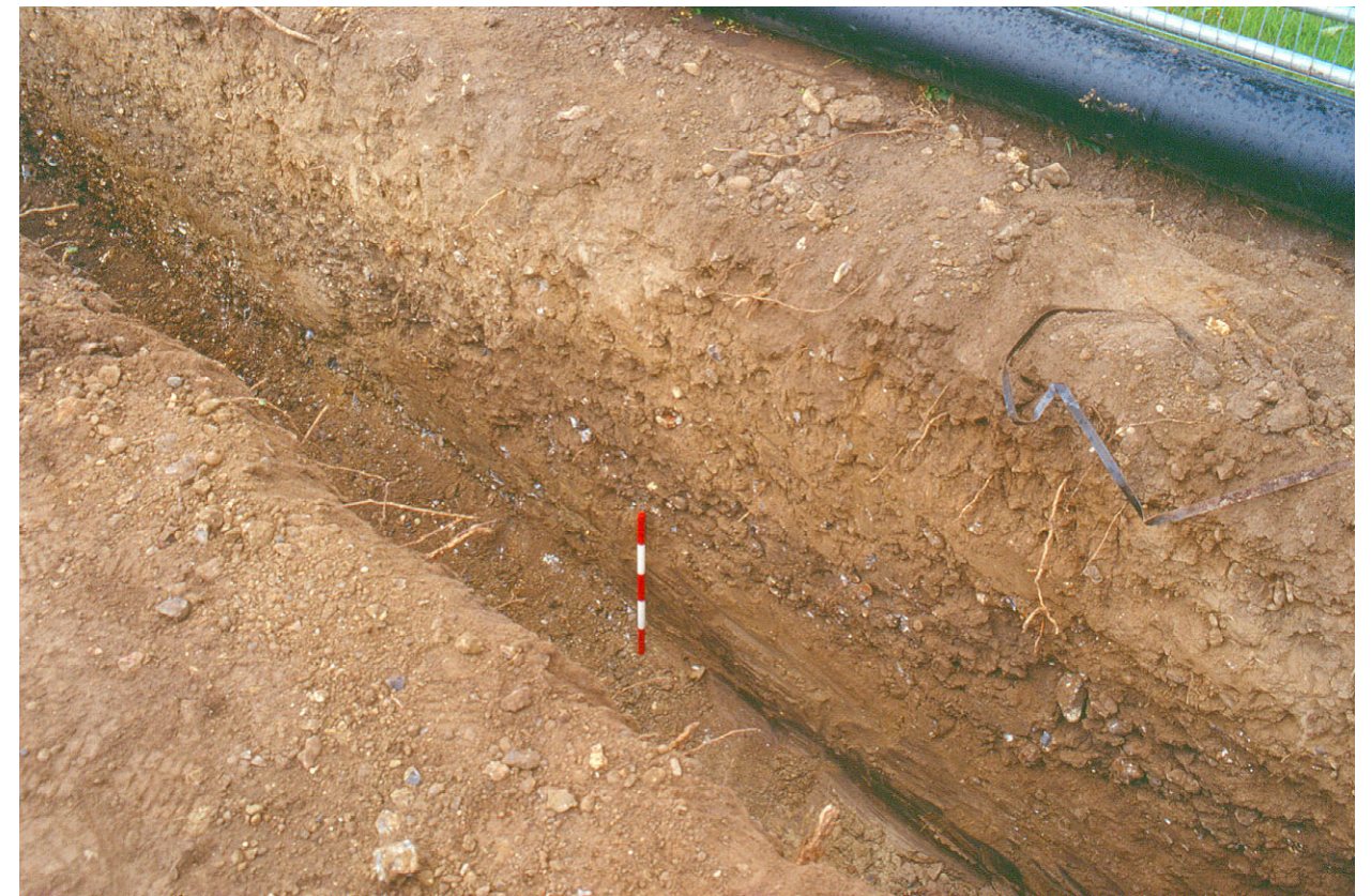
Fig 18 Pipe trench excavation in the playing fields (Area 4 on Figure 15): top left - section just south of the site compound showing the shallow soil horizon and underlying lighter silty (colluvial) deposit, over a former land surface and natural gravel. Bottom left - work in progress. Top & bottom right - views of the fills and overlying deposits in the central and northern parts of the buried stream channel [7] (0.5m scale). The darker waterlaid silt [6] is particularly clear at the base of the lower frame
