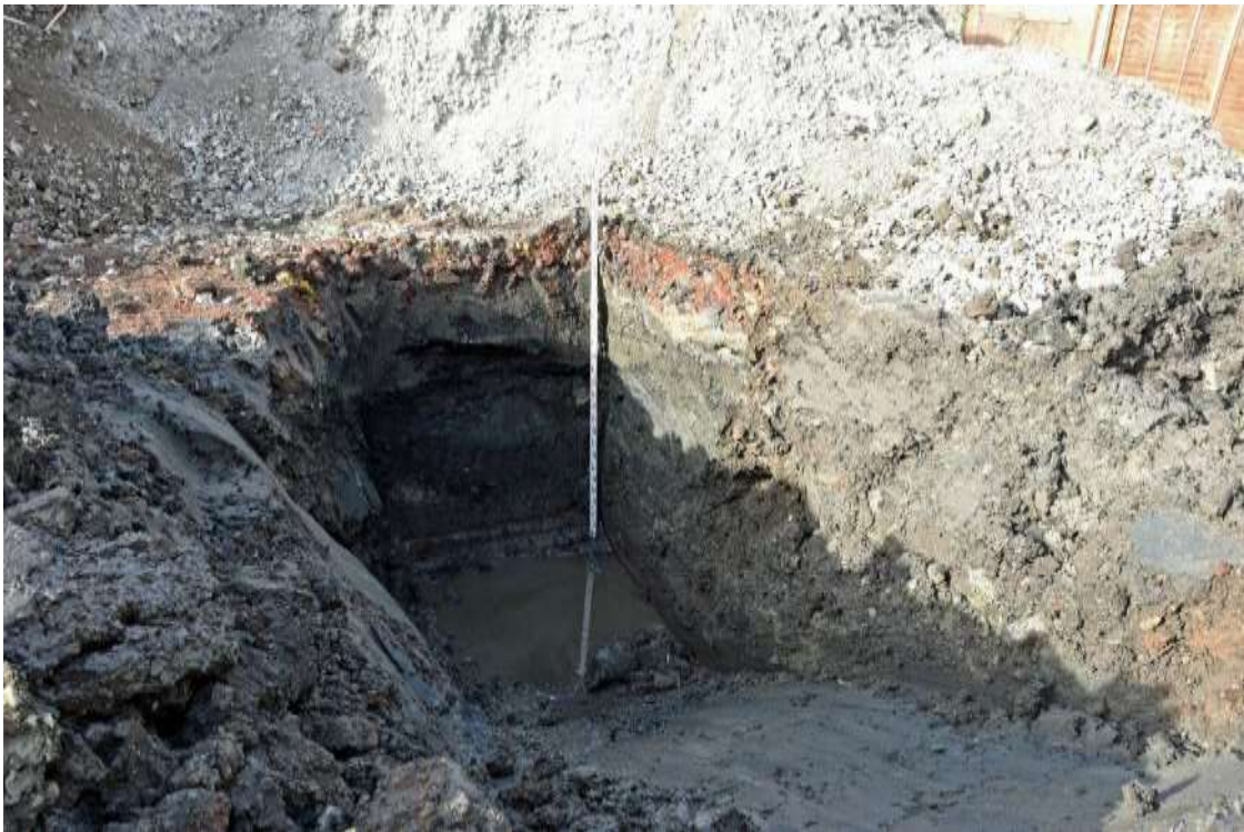
Figure 8: Western end of the completed trench. Facing approximately NW. Scale 3m.
