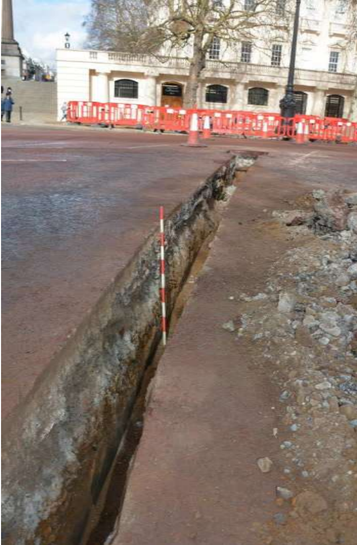
Figure 14: NE-SW trench crossing The Mall. Facing approximately NNE. Scale 1m.
