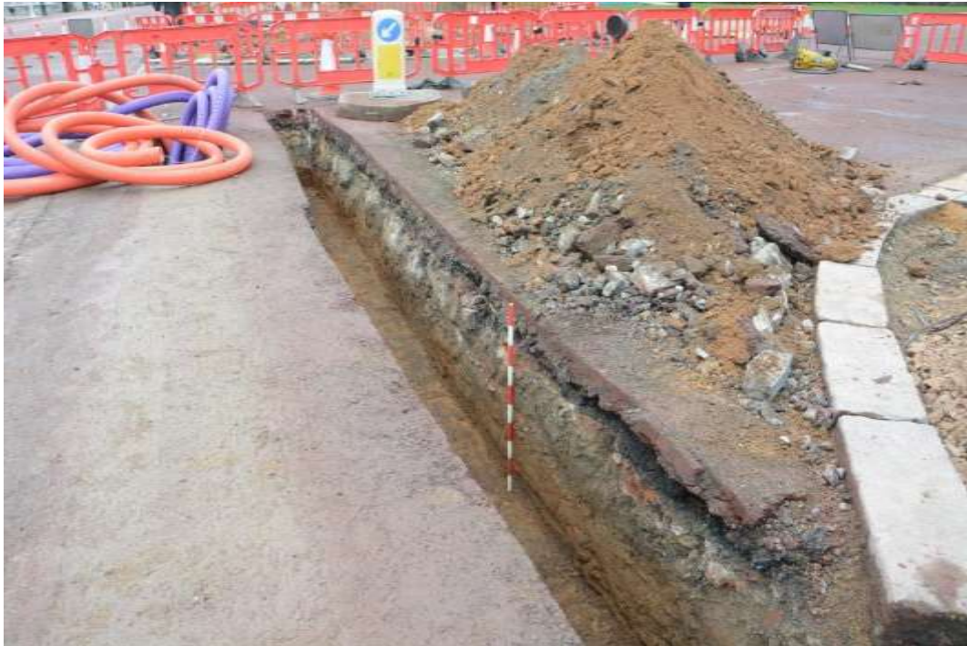
Figure 13: Southernmost east-west trench across Horse Guards Road, showing road make-up and brick rubble overlying natural clean sand. Facing E. Scale 1m.
