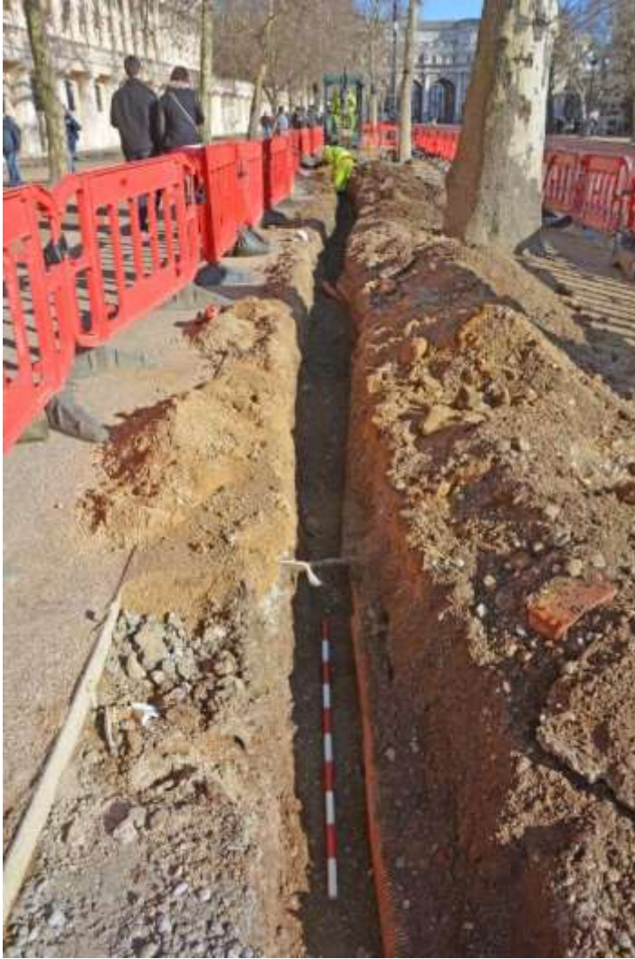
Figure 17: Ducting trenching in North Horse Ride. Facing NE. Scale 1m.
