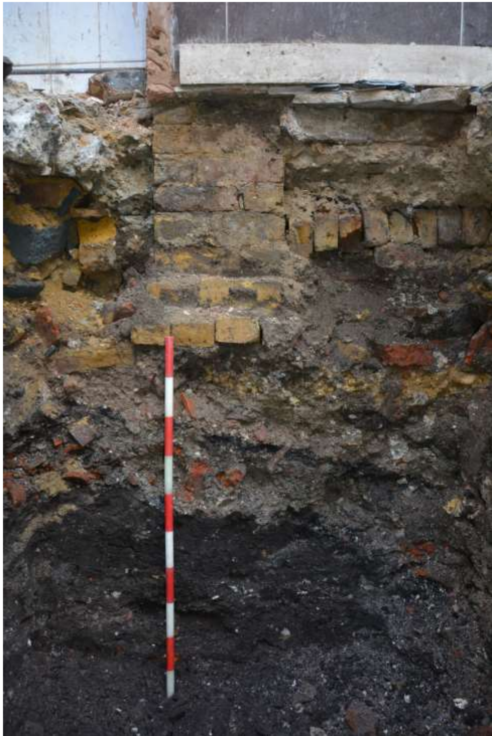
Fig. 11: Detail of the west-facing section of P3: highlighting discrepancy in condition of made ground (24), (25) resulting from above intrusive yellow stock brick wall foundations [23]
