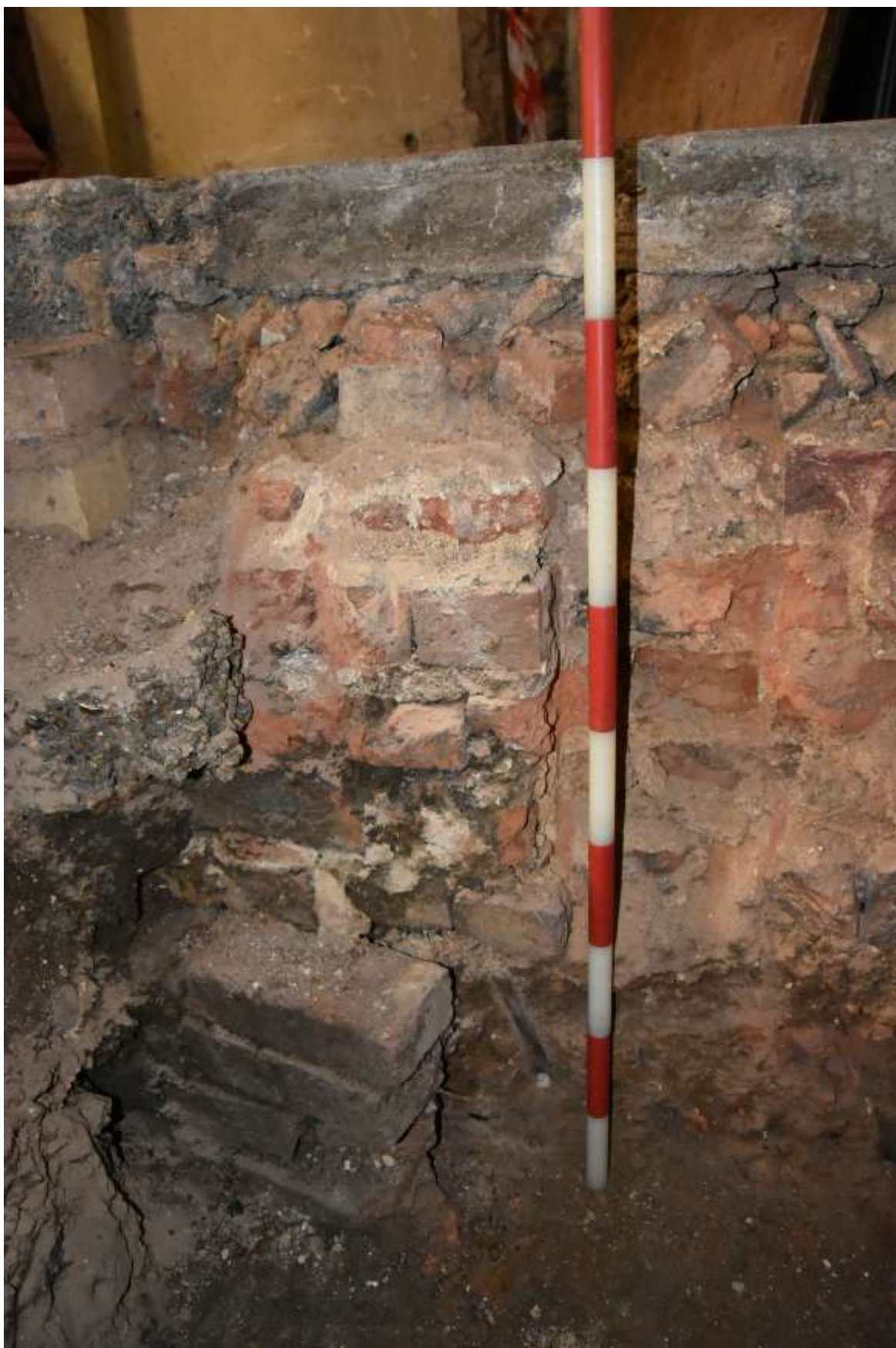
Fig.20: Test pit 1, facing SE, 1m scale. Scale rests in front of wall 8, footing 6 is in the top-left of frame and structure 11 is in the bottom-left of frame. Made-ground (2) is shown in front of 11
