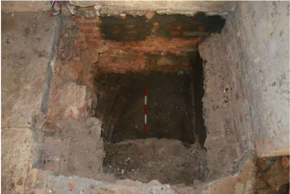
Fig.21: Test pit 1 facing W, 0.5m scale. Wall footing 6 is in the bottom-left corner of the pit, wall 8 is along the left side of the pit. The stepped footings and construction cut [5] are shown across the west, top, of the pit, and the arc of feature 11 is shown in the base of the pit, left of scale
