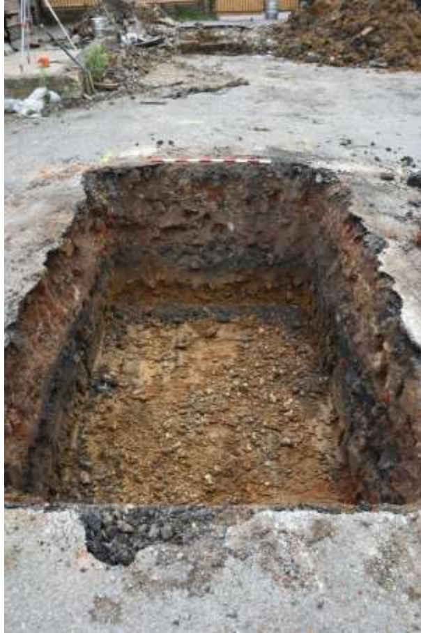
Fig. 20: View of Trench 2 in plan, looking SE (1m scale)
