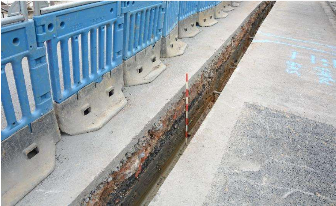
Figure 11: Stratigraphy observed adjacent to Glenfield Terrace. Facing SE. Scale 1m.
