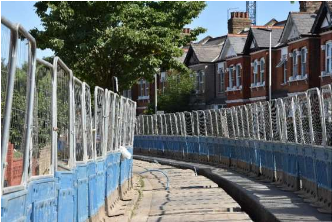
Figure 12: Working shot, looking towards Bonchurch Road. Facing NNE. No scale.
