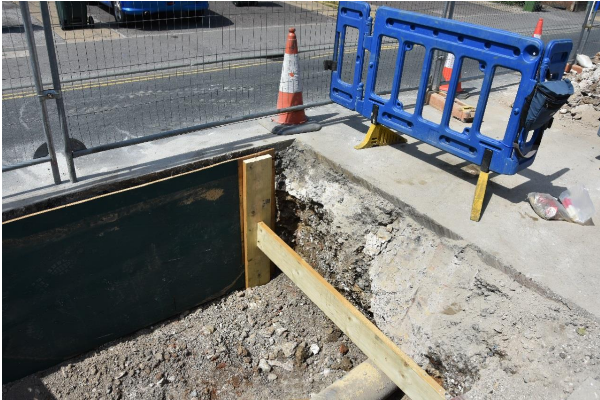
Figure 16: View of timber shoring supporting trench sides, facing NW
