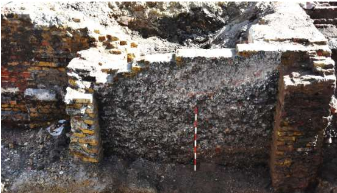
Figure 16: External face of W wall of [205] with tar-like coating. Looking E, scale 1m
