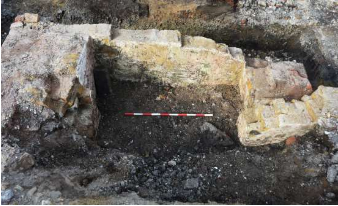
Figure 15: Inside [205]. Note render/paint on inner surface of walls. Looking W, scale 1m
