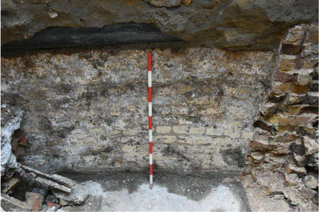
Figure 5: Post-medieval coal cellar observed in the northern section. Facing N, scale 1m.
