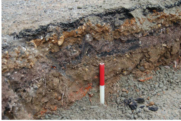
A – Section of gully excavation within tarmac forecourt (0.2m scale).
