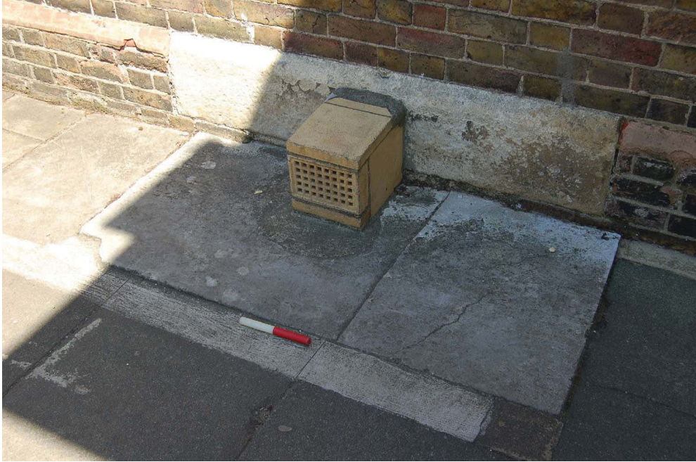
Figure 7: Slab orientated north-south and lain adjacent to the west wall, showing curved upper left hand corner and significant damage including a vent cut through the slab.
