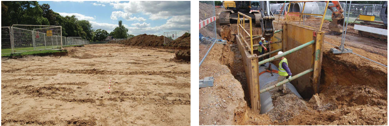
Figure 5: Ground works in Area 3, stripped area and section of pipe trench.
