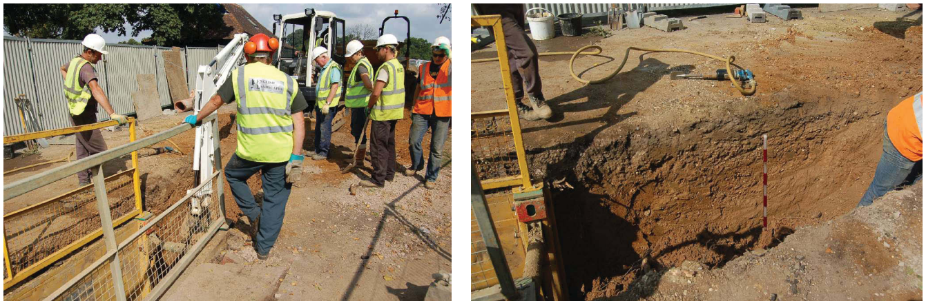
Figure 3: Groundworks in Area 1, working shot and section (east facing).
