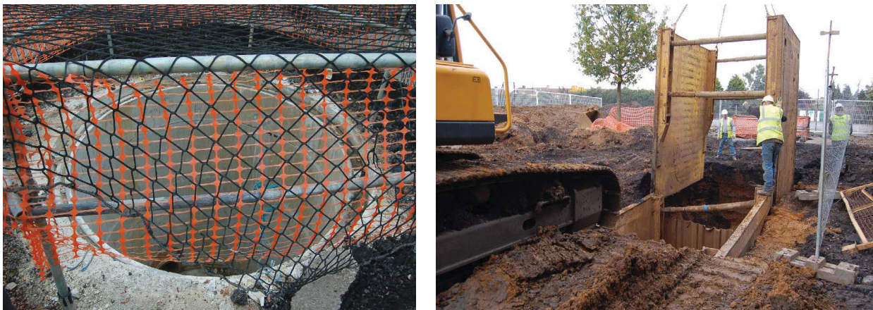
Figure 7: Ventilation column and ground works in Area 5.
