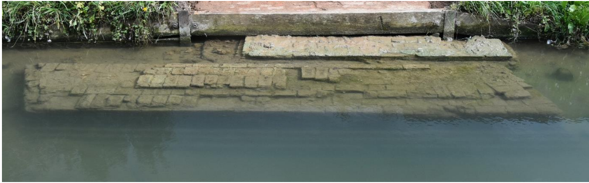
Figure 8: Lower block of waterside bricks in eastern bank. Looking E, no scale. Note three stepped courses visible at base of block.
