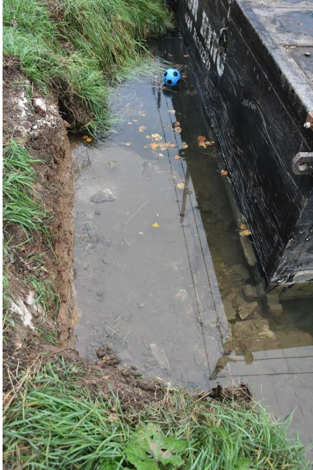
Figure 15: Western footing, post landside portion removal. Looking N, no scale.
