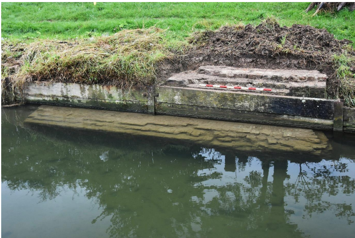
Figure 9: Overall view of footings on western bank. Looking SW, scale 1m
