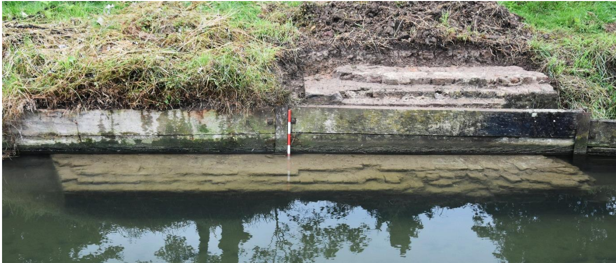
Figure 12: Waterside brick in western bank. Looking W, scale 0.5m
