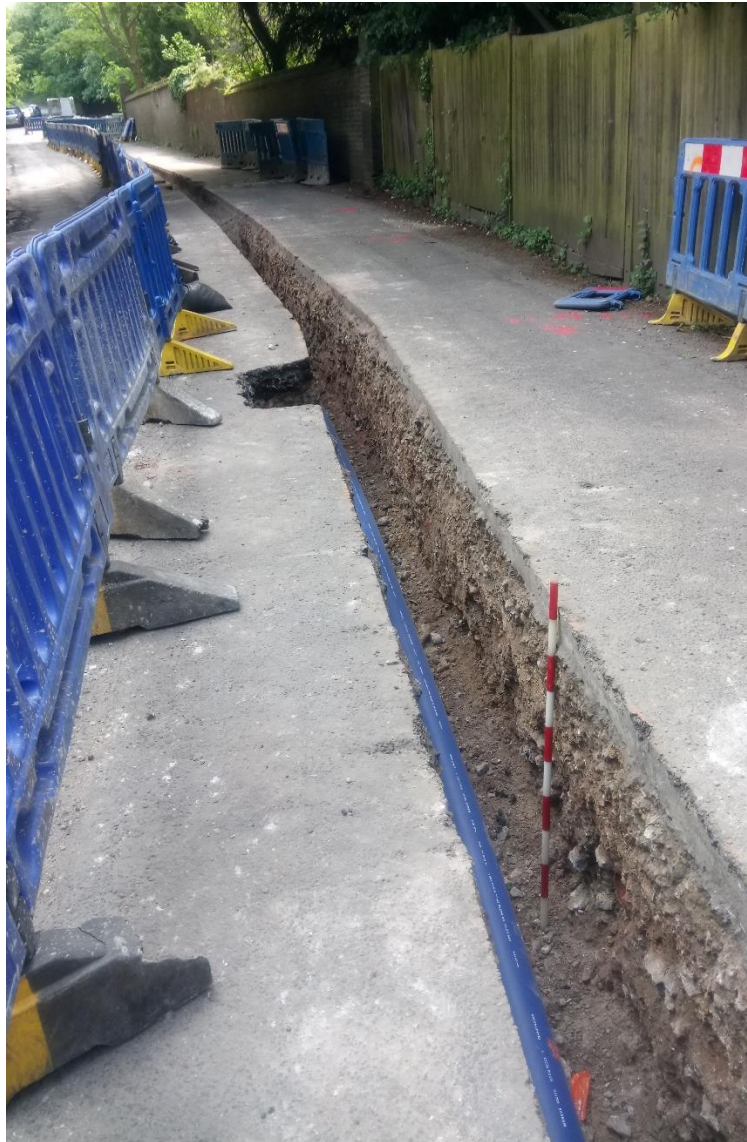
Figure 8: Open cut section of trench, facing SE, scale 1m
